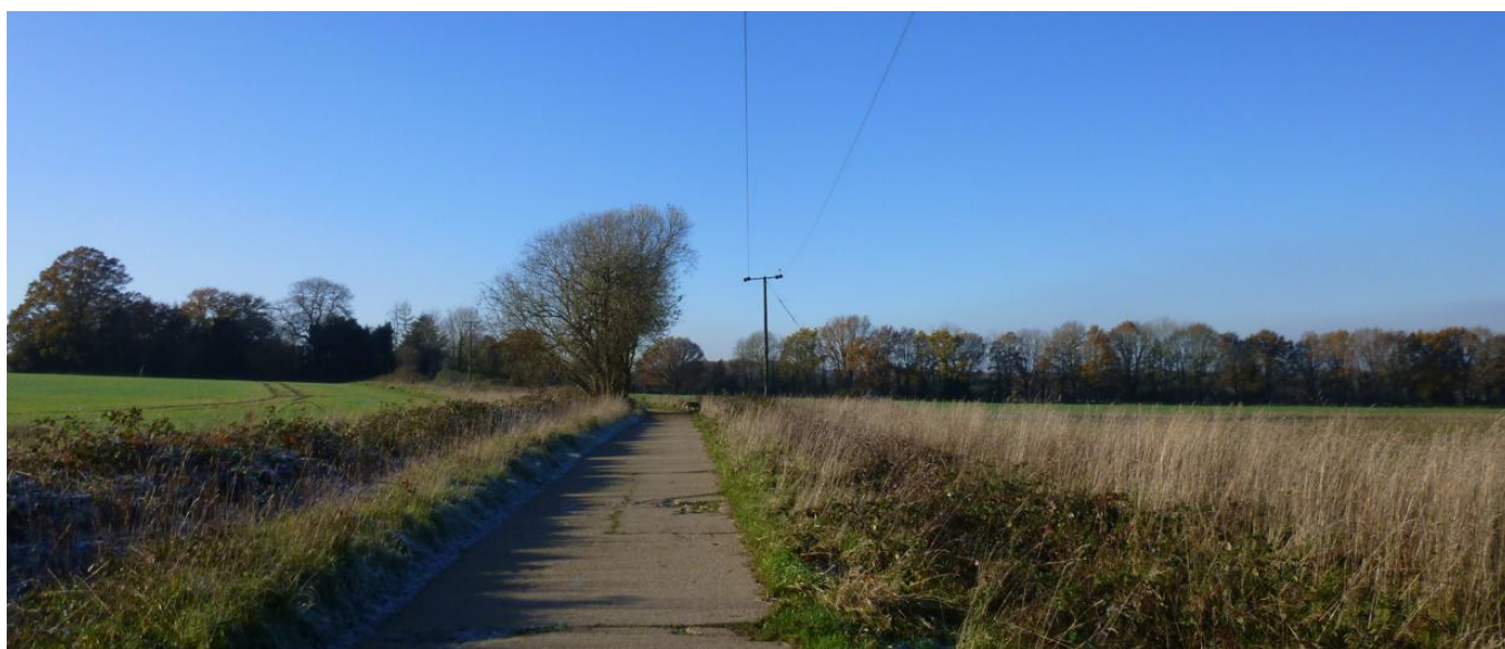
Figure 2 – Overhead HV cable route adjacent to bridleway
