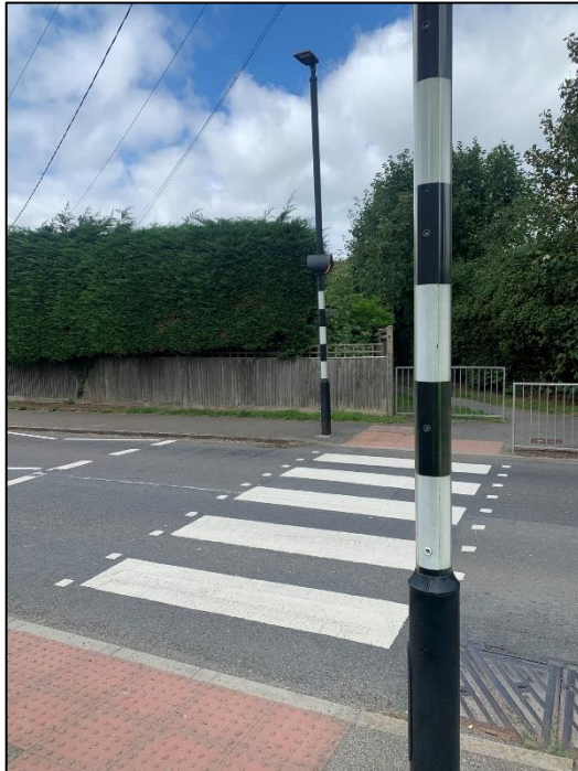
Photograph 6: Zebra crossing along Ardingly Road
