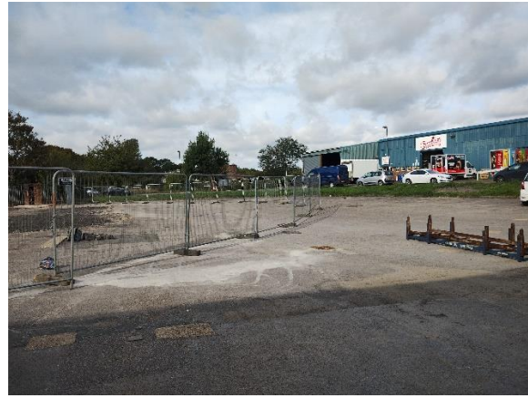
FIGURE 3: EXISTING SITE FACING NORTH WEST
