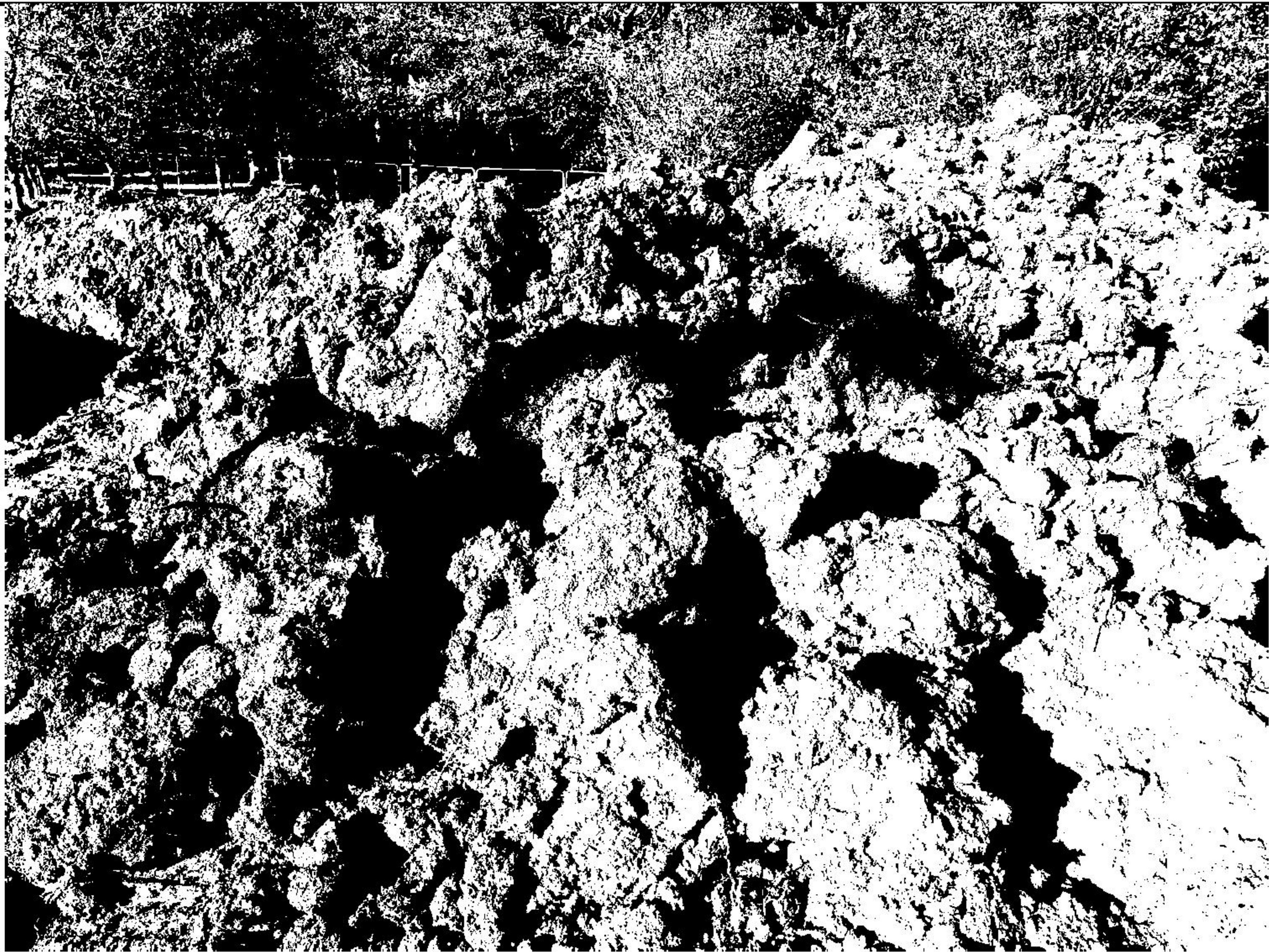
Plate 6 - Overview of subsoil stockpile SSP1 after additional subsoil placed (Dated 21.11.2025)
