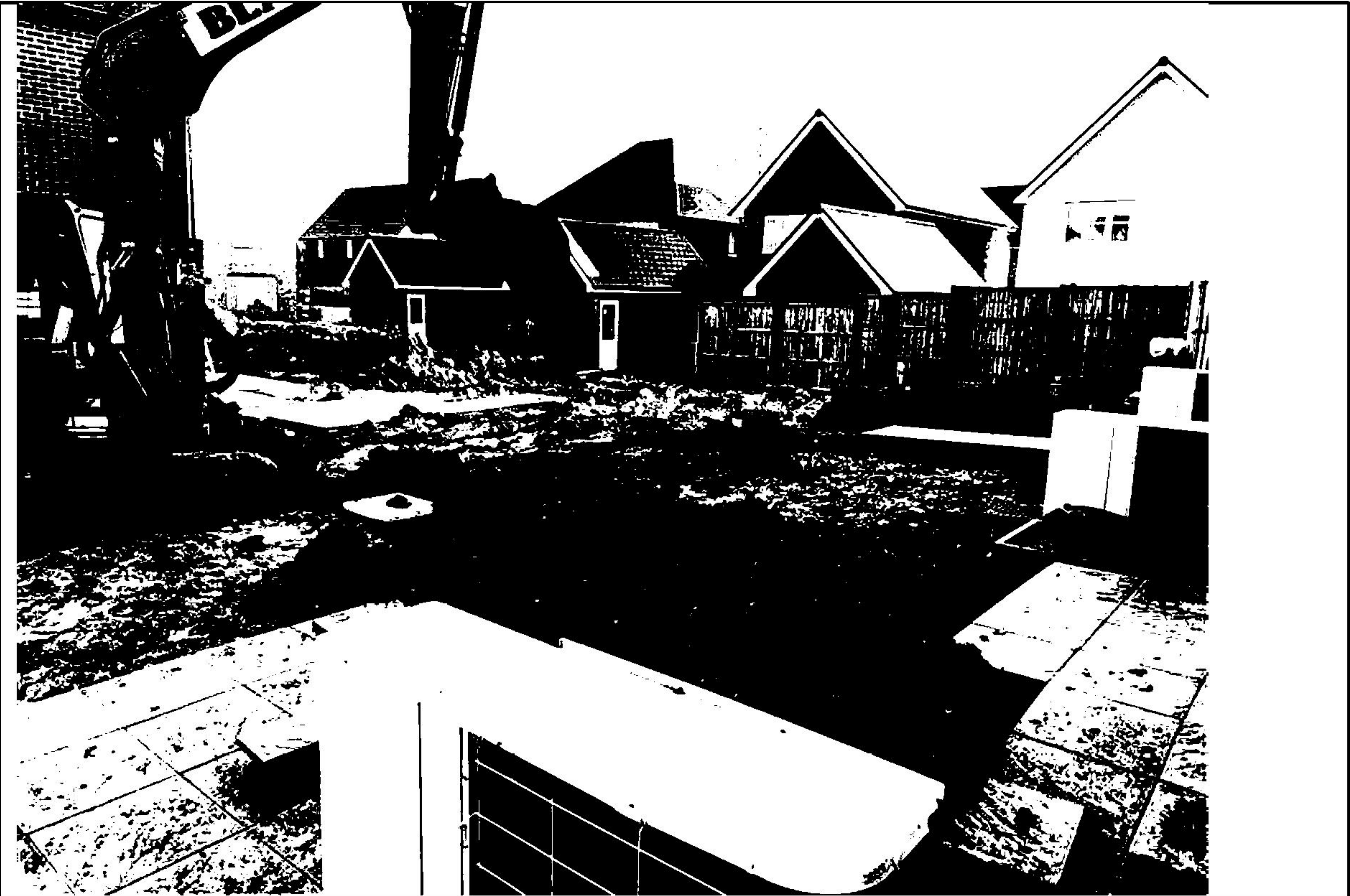
Plate 11 – Overview of topsoil being placed in Plots 3, 4, and 5 (Dated 03.12.2025)
