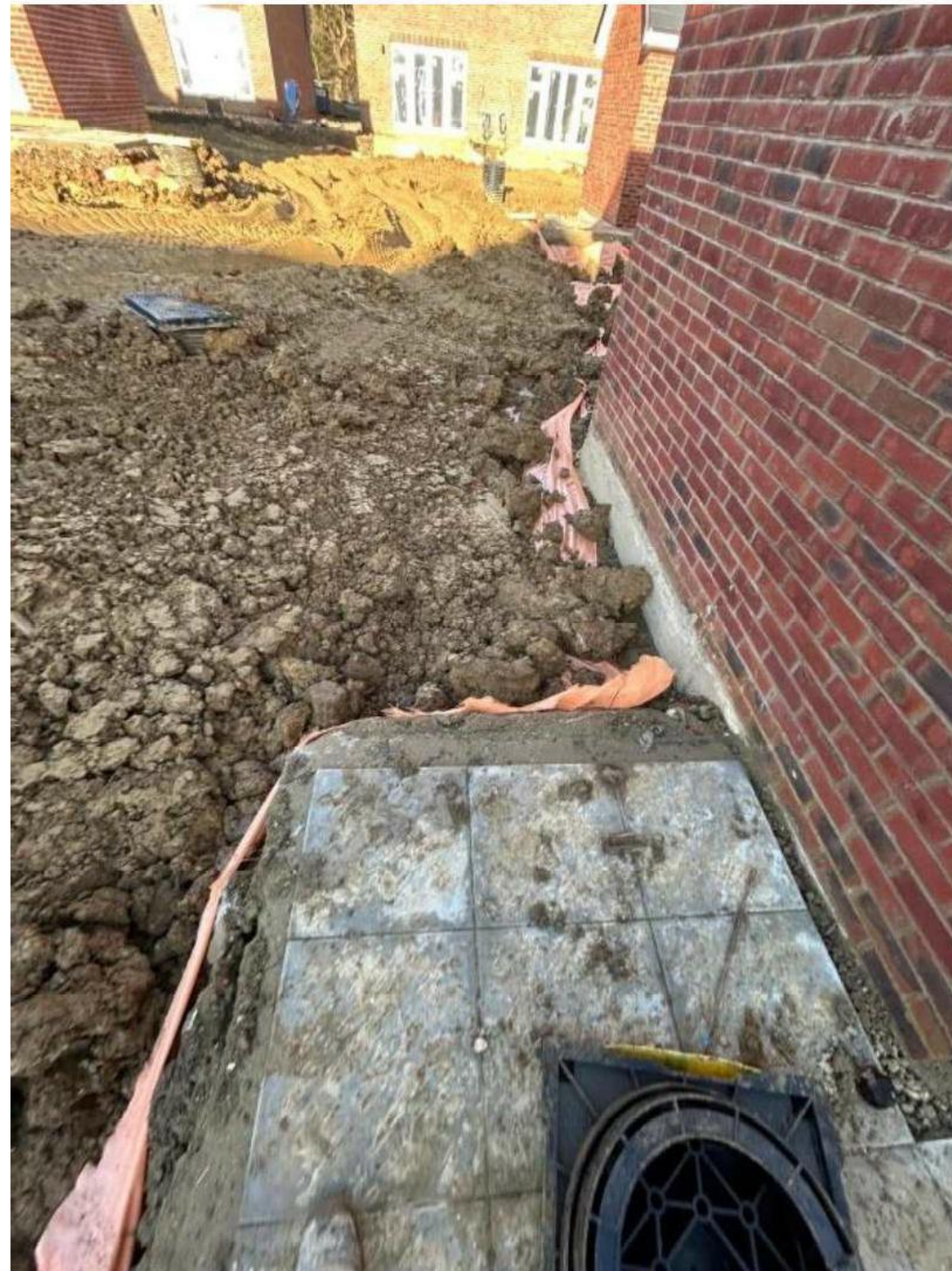
Plate 27 – Photographs of membranes being installed within Plot 3-5, Plot 34
