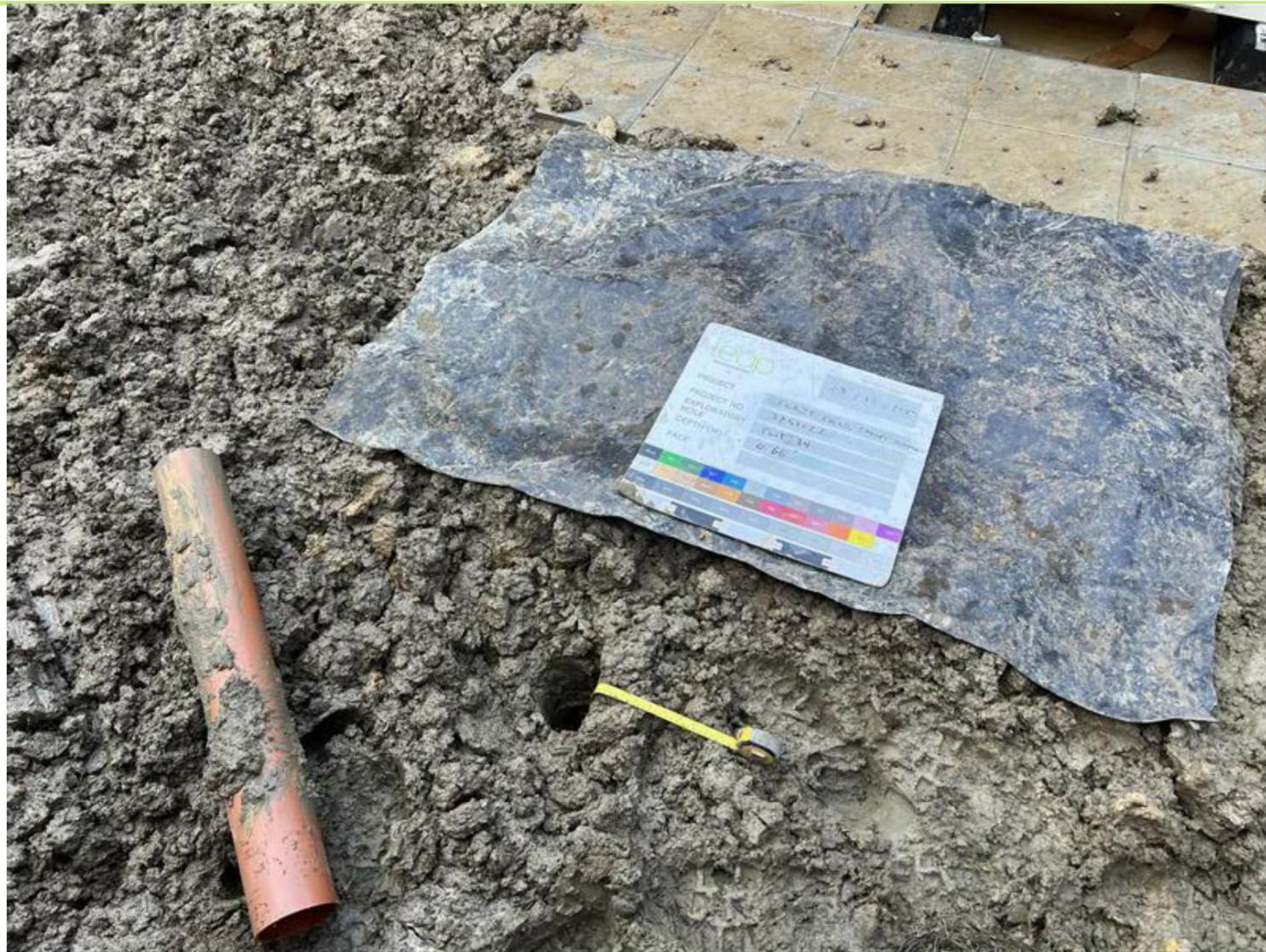
Plate 25 – Overview of Plot 34 inspection pit (Dated 03.12.2025)
