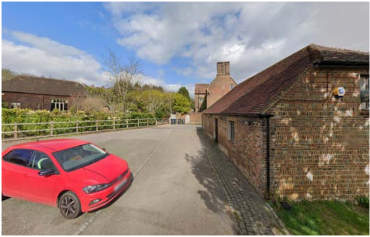
Existing building in Hurst Grange Photo 5
