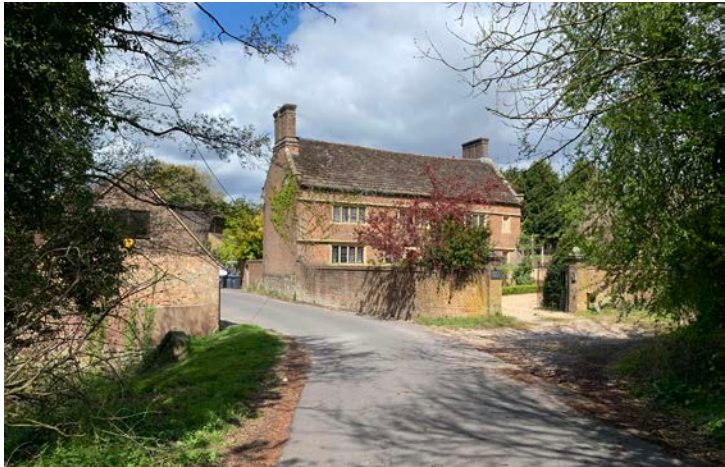
Hurstwood Grange access from Hurstwood Lane Photo 1
