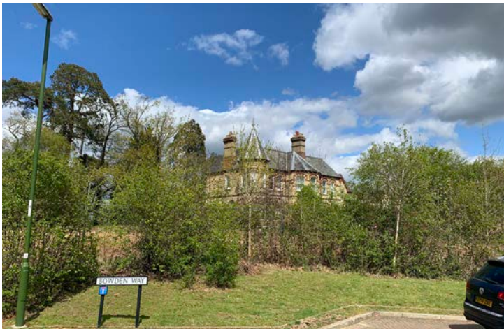
View to existing building behind Bowden Way
