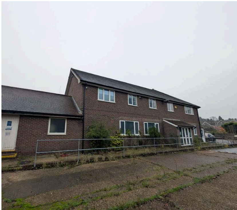
Figure 9. View of B1 on site (taken November 2024).
