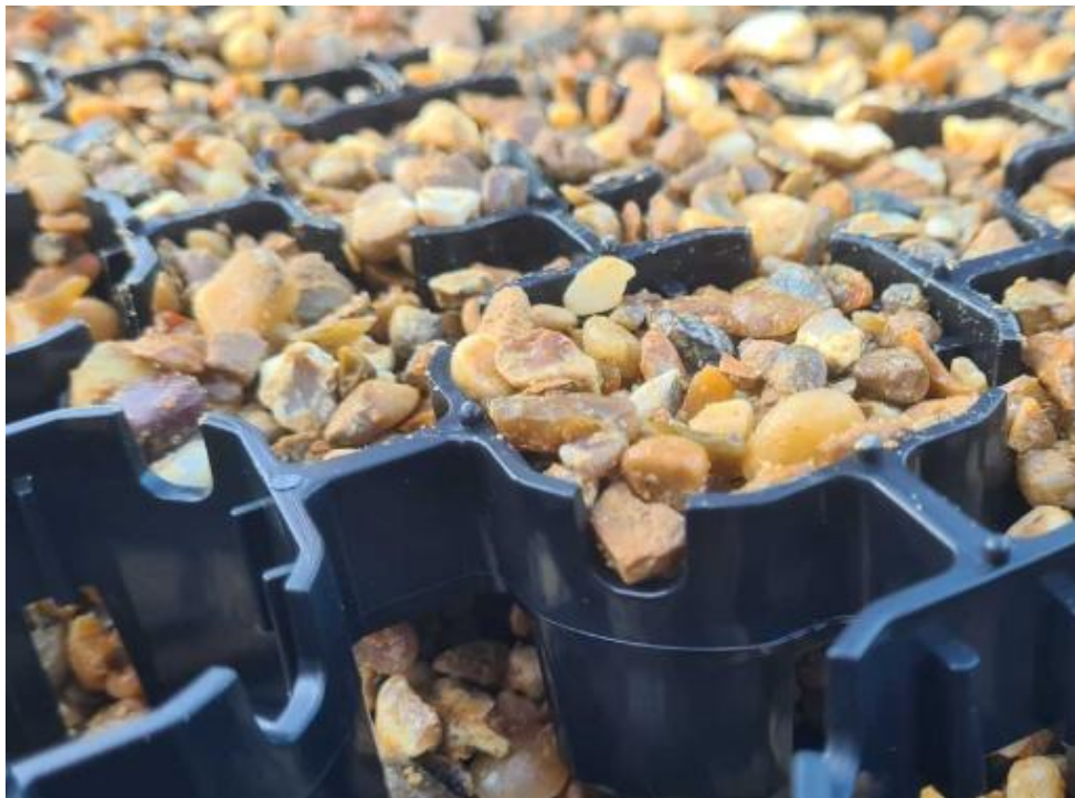
Appendix 13 – Example of the golden pea gravel proposed for the widened driveway, selected to match the gravel already used throughout the original Barnfield development.
