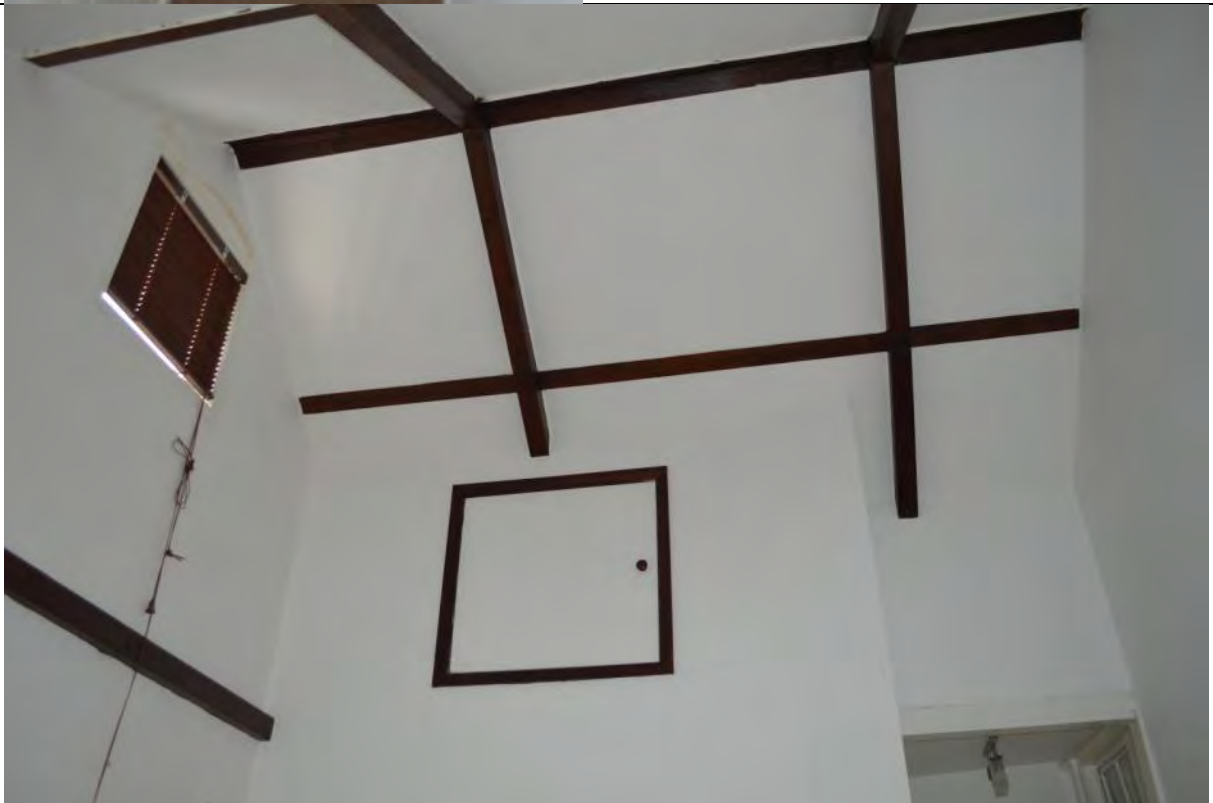
Plate 14: Interior of the southern room in block 1
