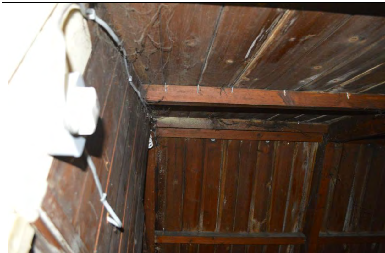
Plate 15: Interior of the matchboard lined roof structure over the central bedroom (block 1) and the matching partition between the central and northern room in block 2
