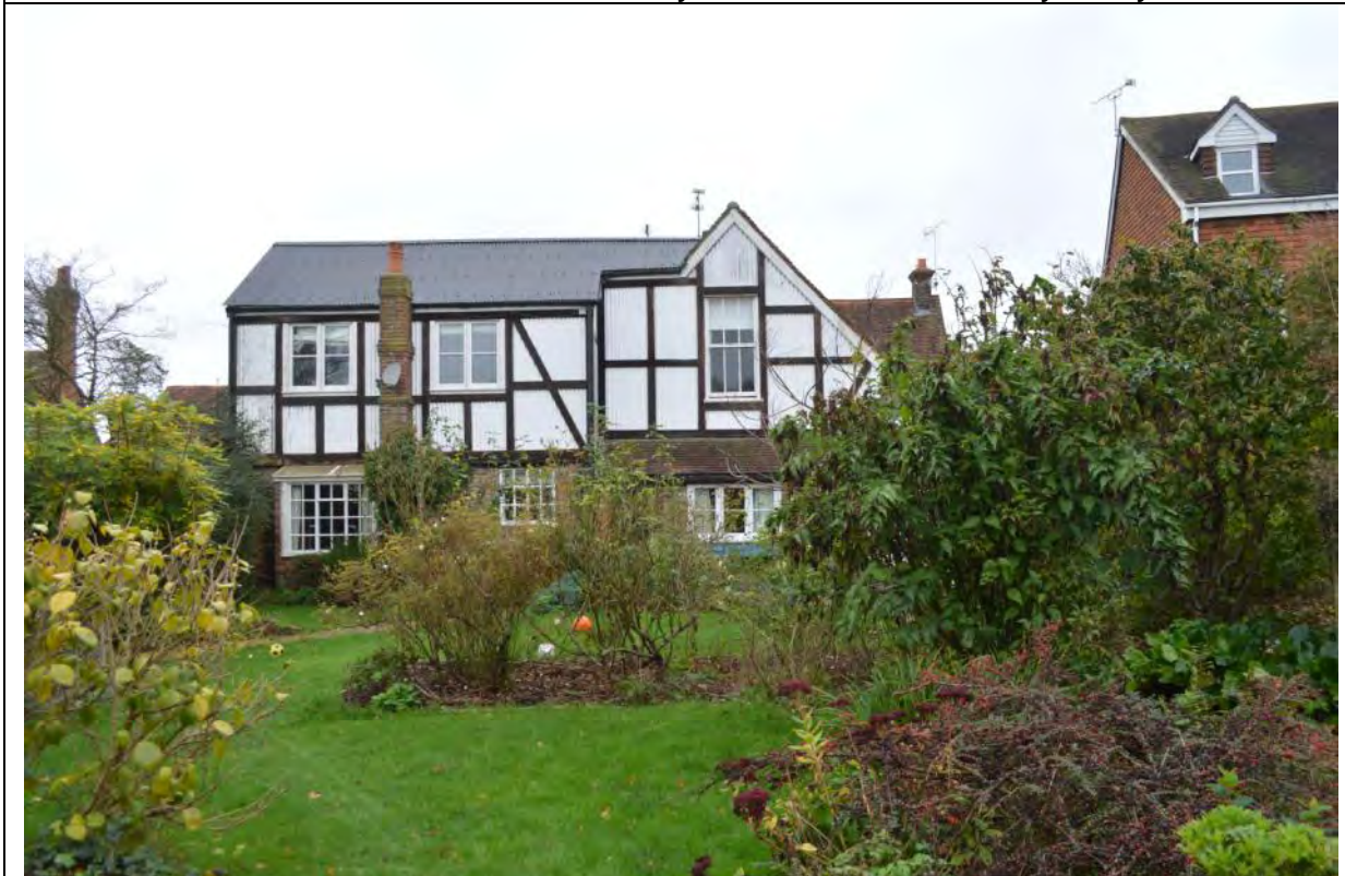
Plate 4: The principal, east – facing elevation
