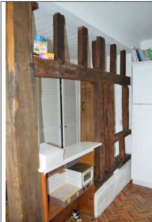
Plate 9: Timber framed wall in the current kitchen (cross-wing, block 2), viewed towards the rear (west) of the house
