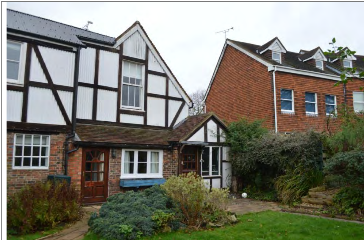
Plate 5: The north end of the east elevation (the face-wing, gabled extension and lean-to)
