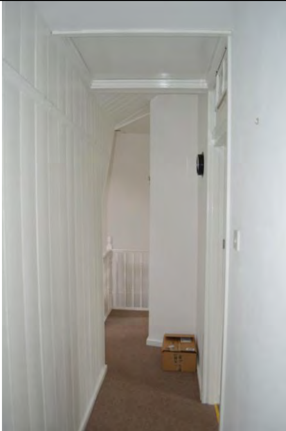
Plate 13: The corridor looking north, note matchboard to the west with picture rail and plain-finish to the inserted corridor wall on the east
