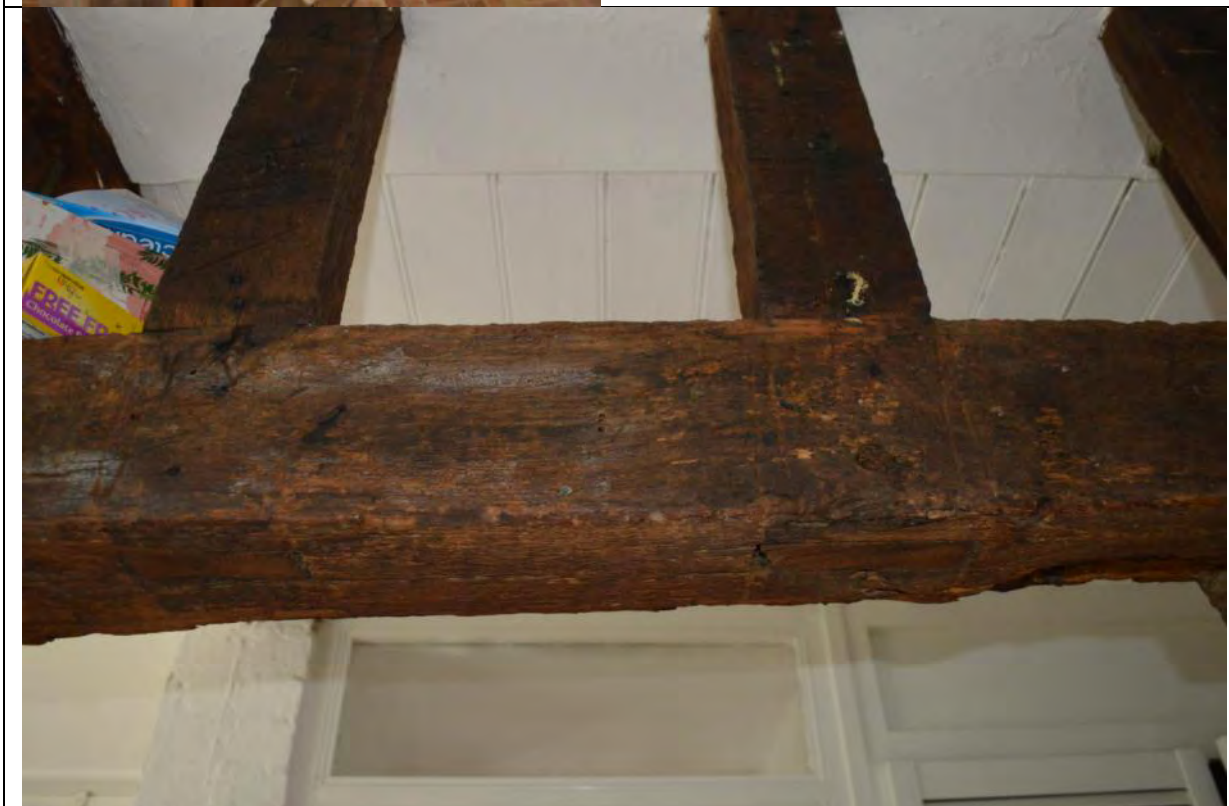
Plate 10: Details of the mid-rail with in situ studs above and mortises on the same alignment below, note that the studs are flush with the mid-rail
