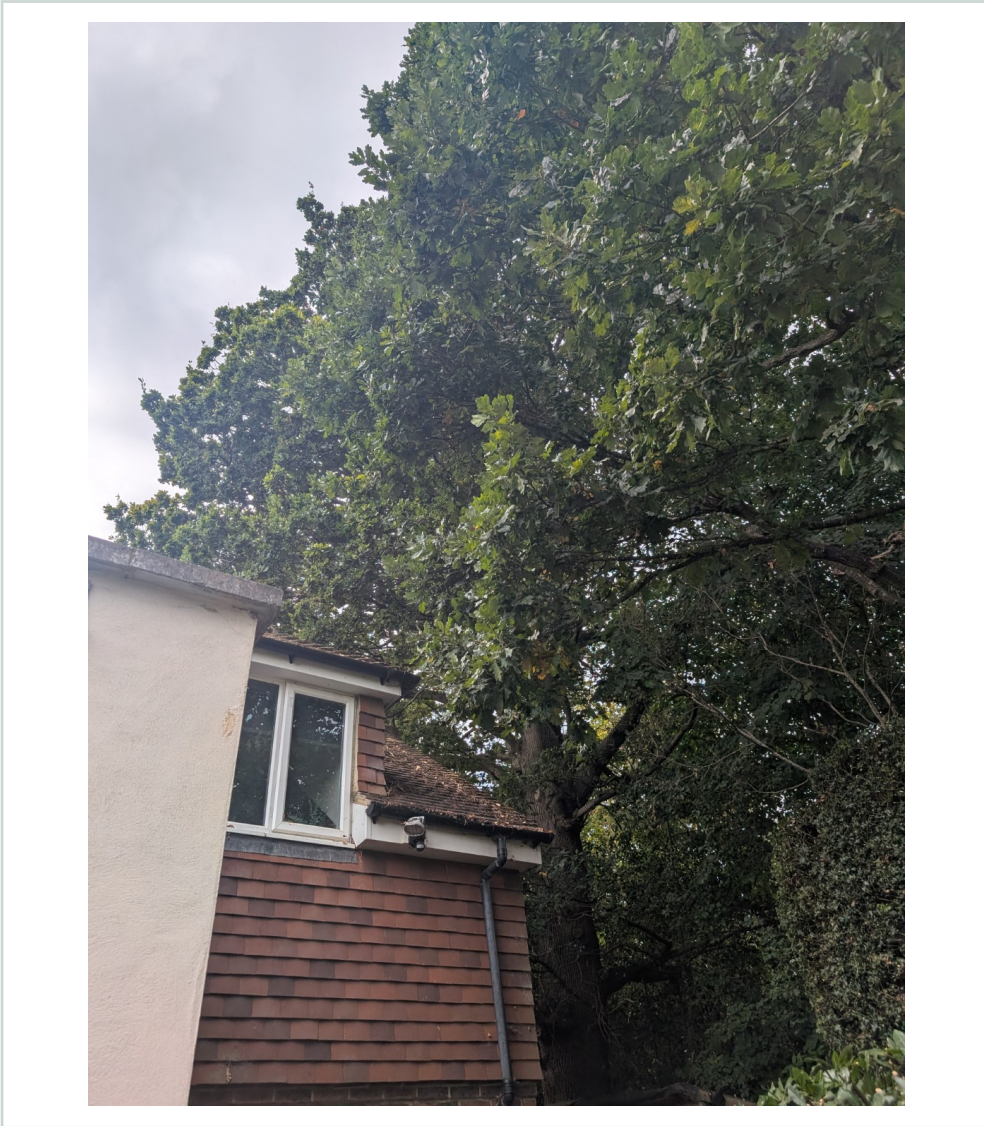
E3 Oak canopy close to main house roof
