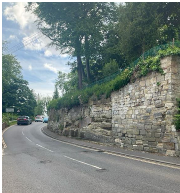
Photograph of retaining wall to be repaired
