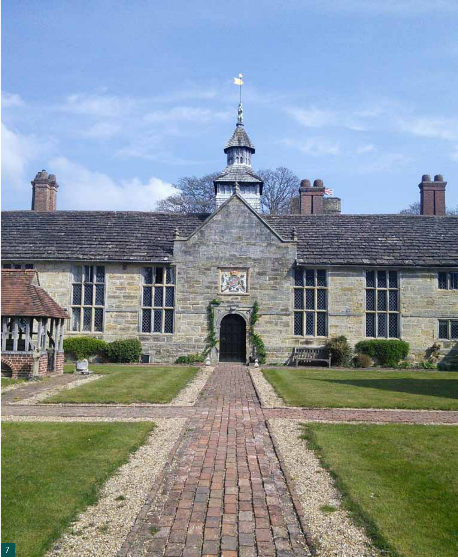
7 Photograph of internal courtyard area at Sackville college
