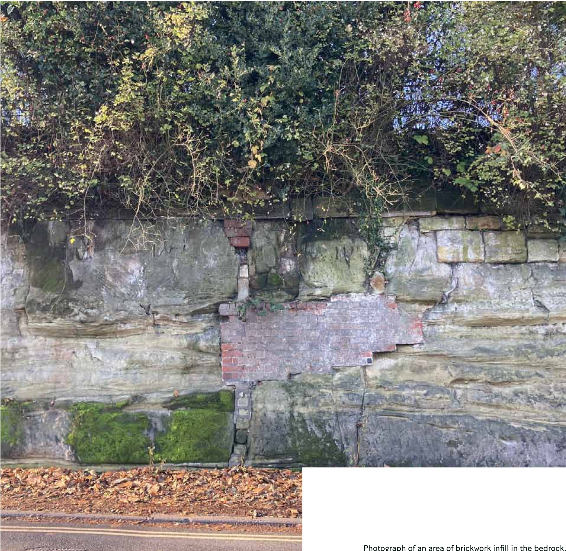
Photograph of an area of brickwork infill in the bedrock.
