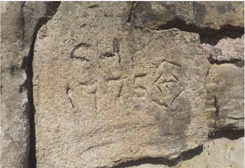
Wall Date Stone
