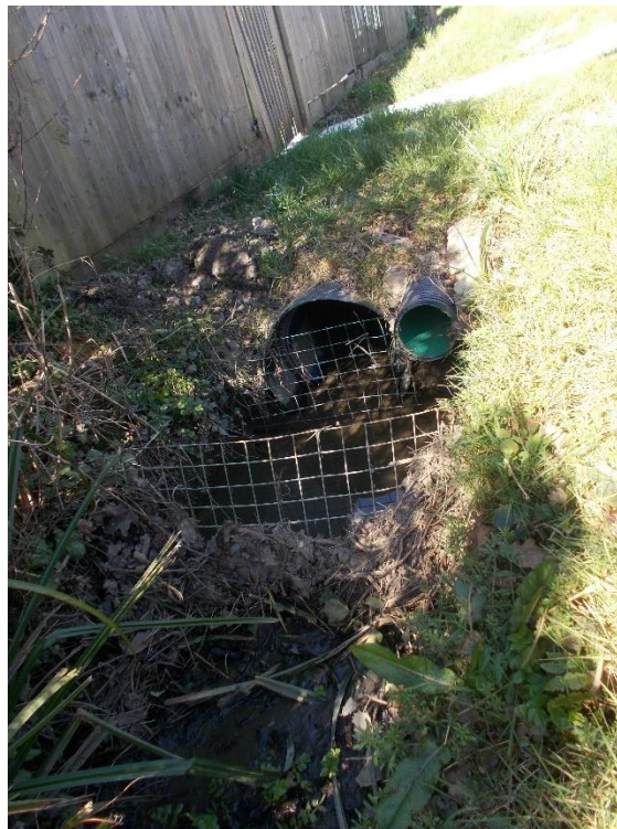
Culvert in Truslers Hill Lane
