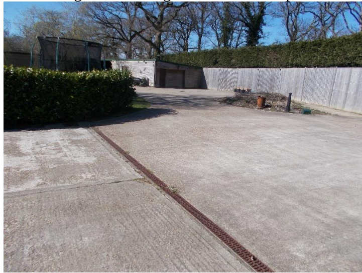
Parking area showing surface water strip drains
