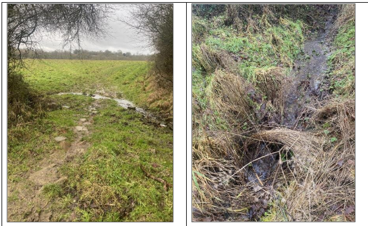
Figure 2-6 (Left) Drain 1 in the north (right) Drain 8
