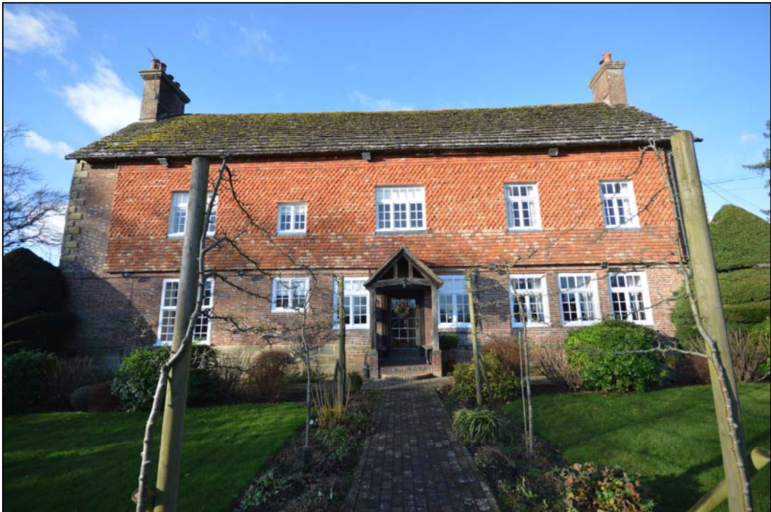
Plate 3: The principal east-facing elevation of the east wing showing the brickwork and the tile-clad timber-frame
