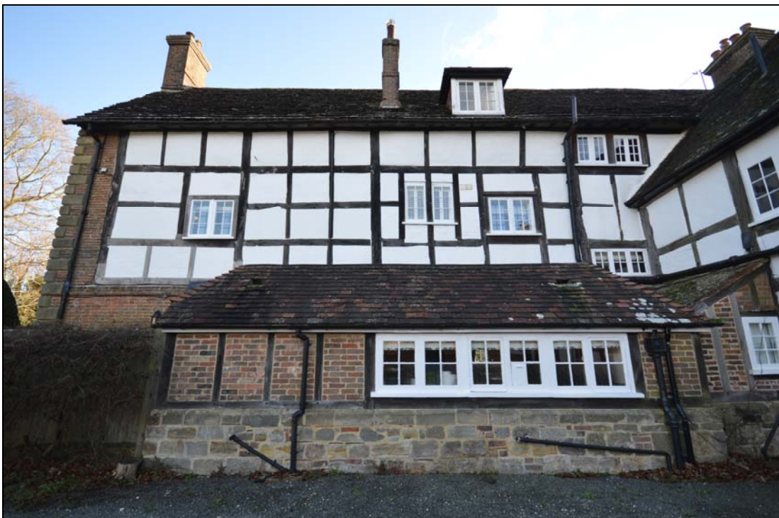
Plate 8: The rear (west) elevation of the wing showing the 20 th century lean-to extensions
