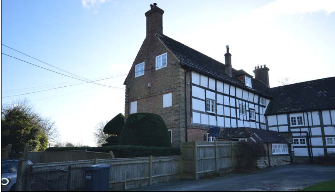
Plate 4: The north and west elevations of the east wing showing the different materials used in the building's constructions and the modern lean-to extensions
