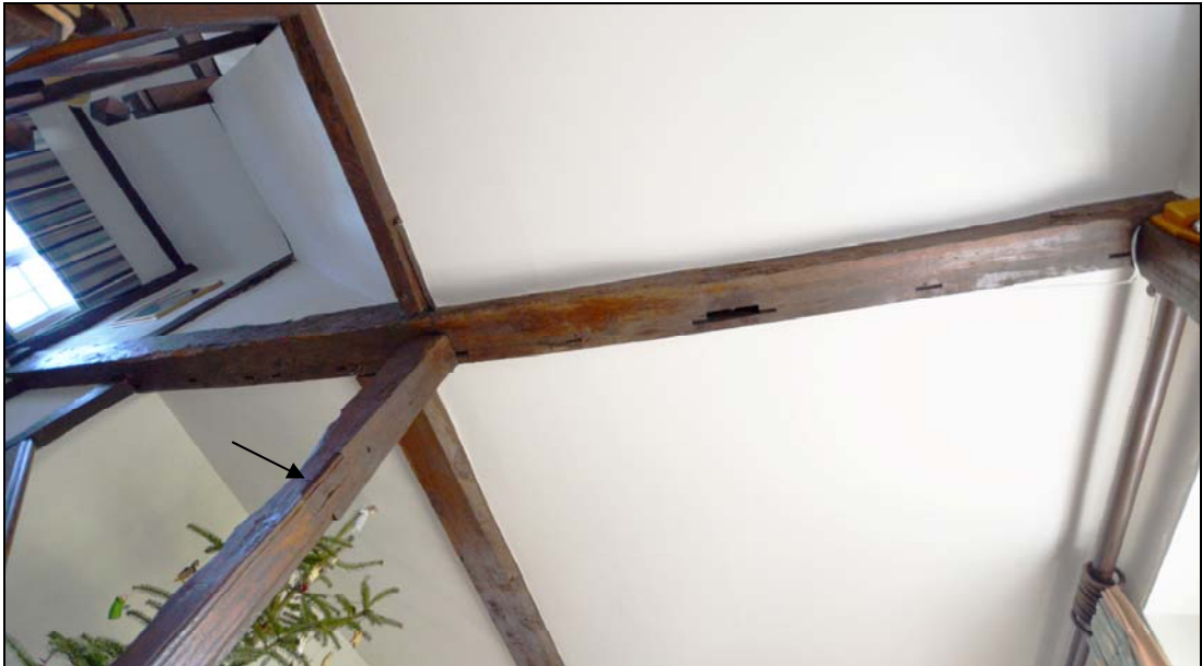
Plate 6: Soffit of the cross-beam between bays 1 and 2 with jointing for a partition and a doorway, the mortise for the head plate of the door can be seen in the post (arrow). Note also that the partition had continued to the west side of the building enclosing the staircase
