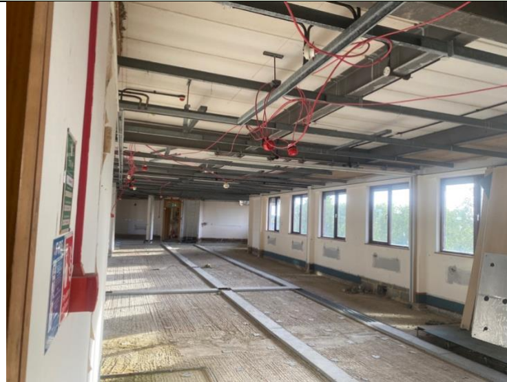
B1: third storey room on northern elevation
