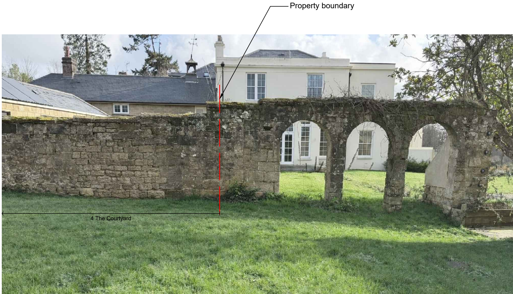
View of existing wall
