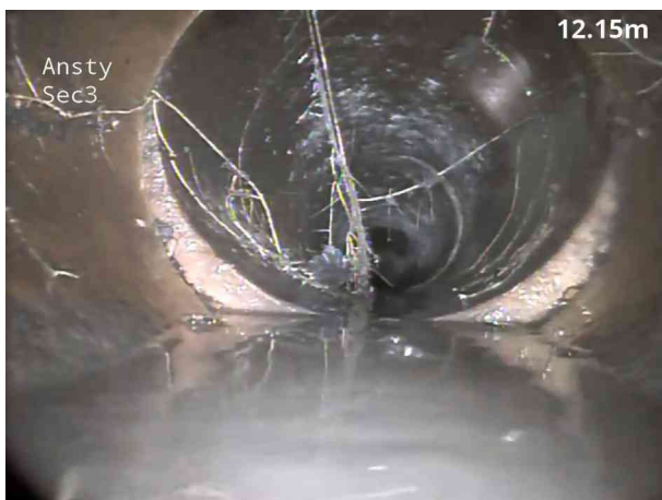
9, 00:01:44, 12.60 m Junction at 2 o'clock, 100mm dia
