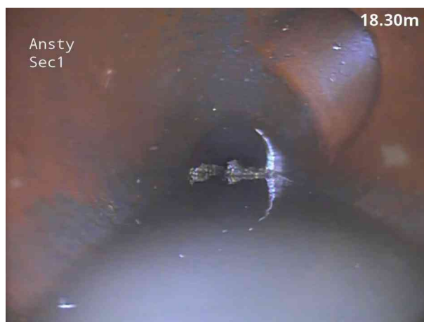
10, 00:02:08, 18.40 m Junction at 2 o'clock, 100mm dia
