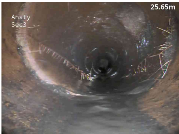
13, 00:02:42, 26.00 m Junction at 2 o'clock, 100mm dia
