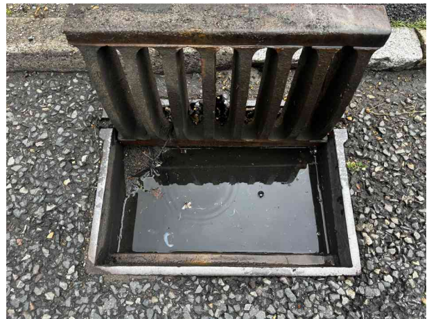
RG adjacent to hard stop, high water level
