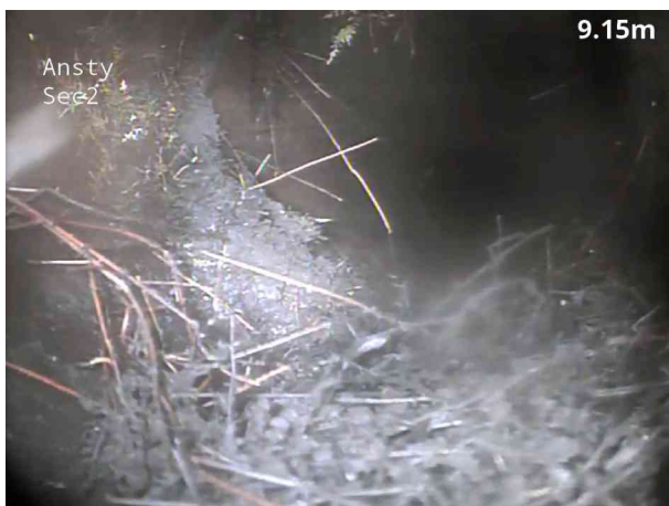
15, 00:01:52, 9.20 m Roots, mass, 10% cross-sectional area loss, change
