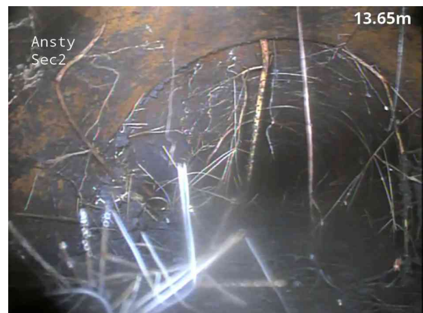
18, 00:02:12, 13.80 m Roots, mass, 40% cross-sectional area loss, change
