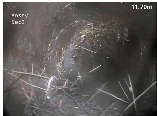
16, 00:02:01, 11.80 m Roots, mass, 20% cross-sectional area loss, change
