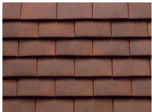
Clay roof and hung tiles
