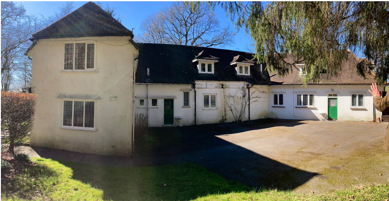
3.3.1 / i Existing Lodge/ east view
