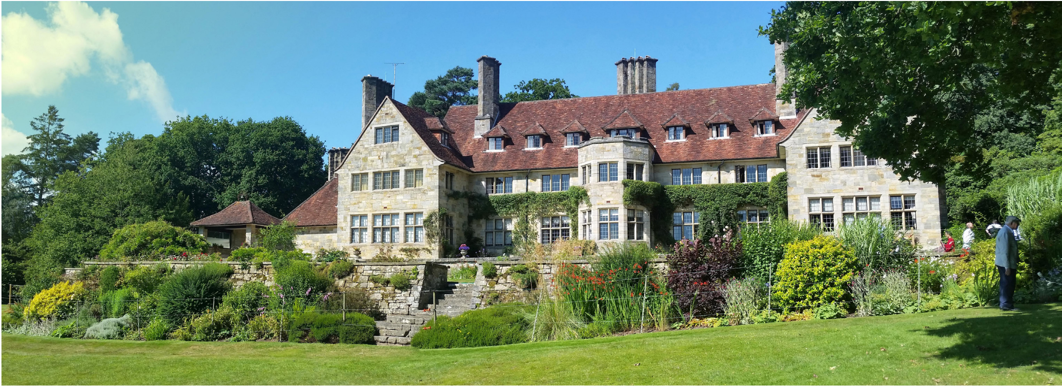
3.2.9 / i Existing Manor
