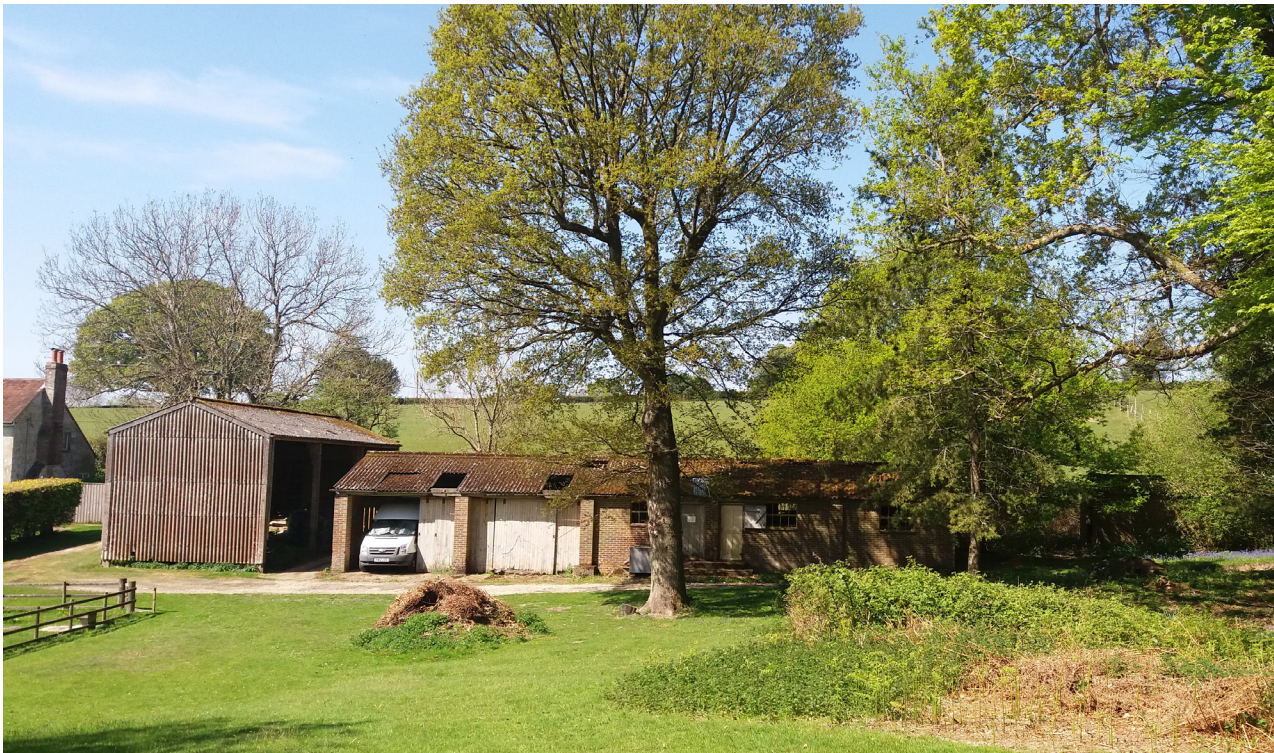
3.4 / ii Existing Stables
