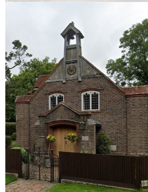
Ansty Village - Formerly St John's Chapel (now a house)
