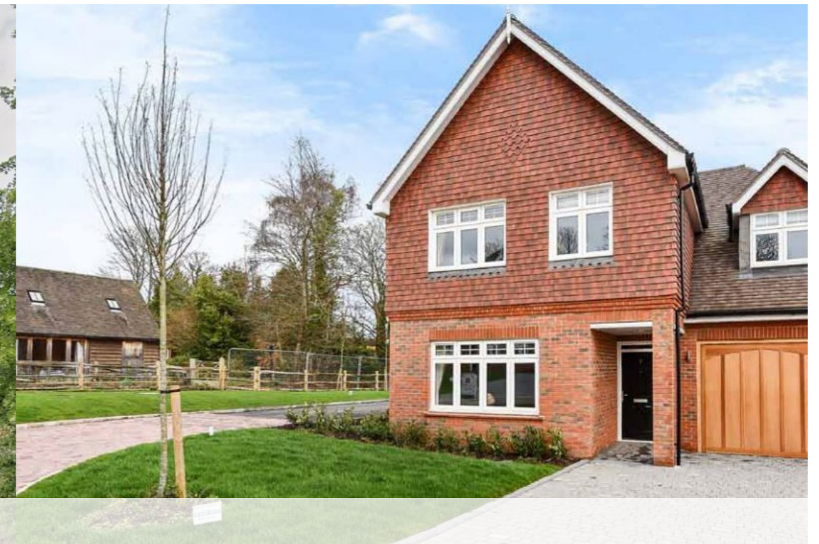
Brickwork banding and detailing - at material transitions
