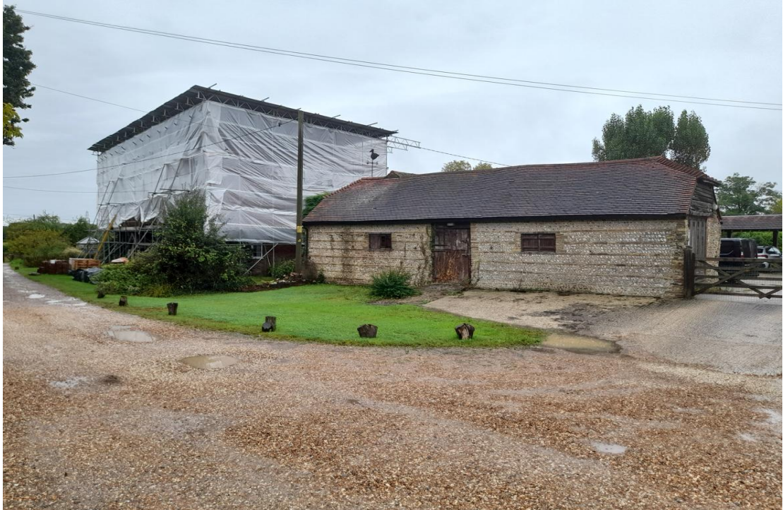
Fig. 8: View, looking north-west from Gratten Lane, of the flint farmstead building and the Farmhouse.
