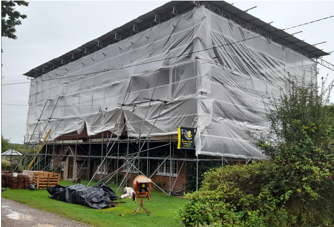
Fig. 6: View of Wyndhams Farmhouse, looking north-west, with protective scaffolding and covering.
