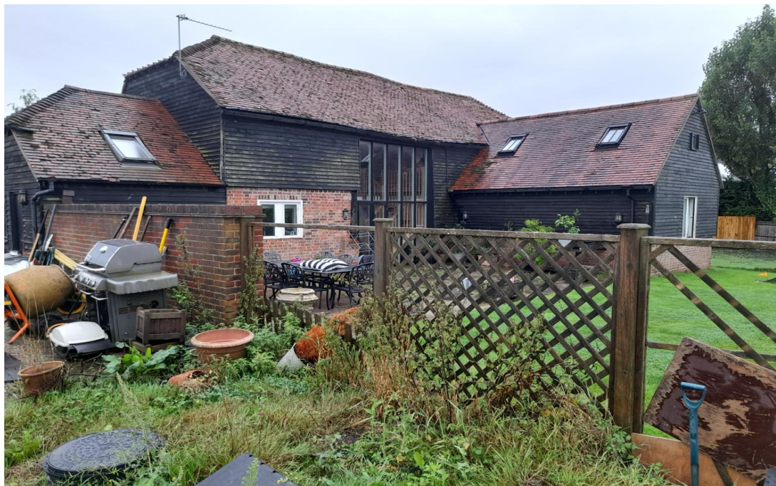
Fig. 9: View, looking south-west, of the rear elevation of the converted former barn.
