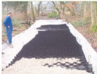
CellWeb during installation.
