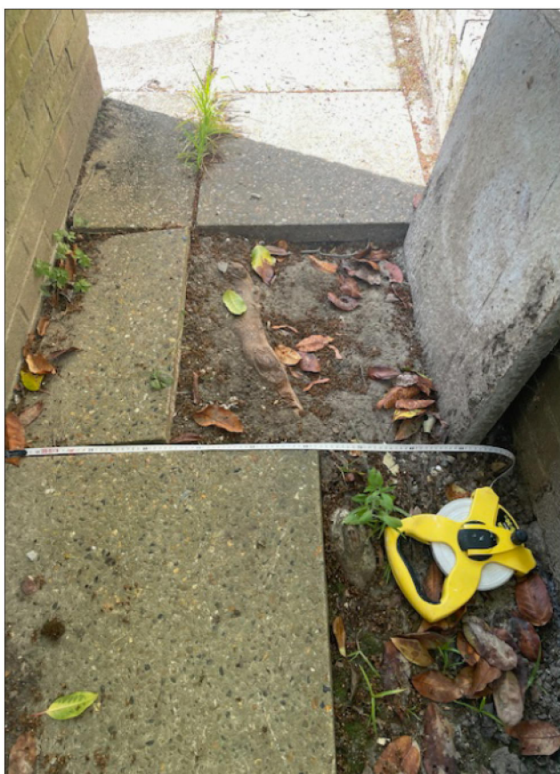
Fig. 2: Roots growing alongside existing structure to be covered with suitable ground protection during demolition and construction phases.
