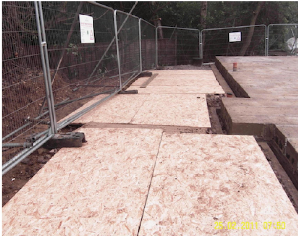
Fig. 1 Heavy duty boards over sharp sand and wood chip
