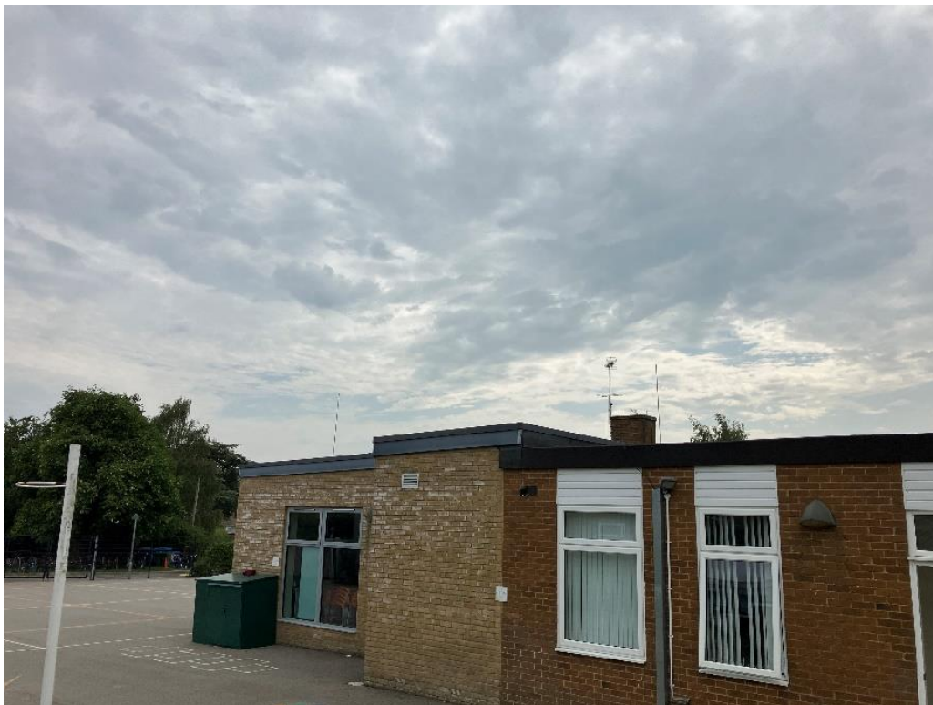
4.8: Image 6 - Ground view from West of building
