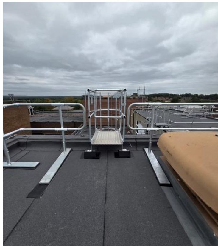
6.2: Image 2: Example image of CAT Ladder junction with guardrail
