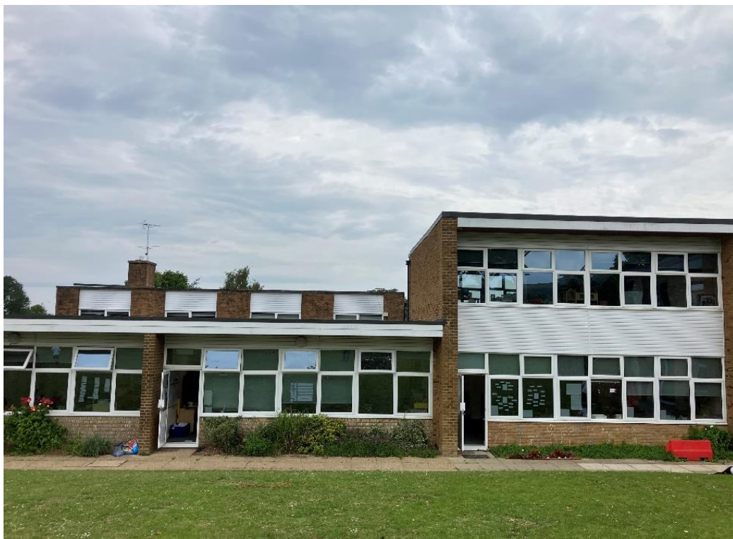
4.6: Image 4 – Ground view from South of building
