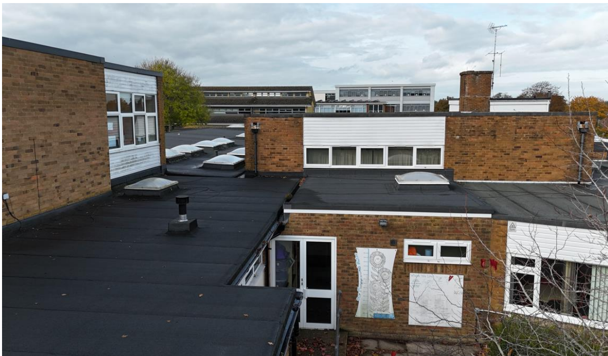
5.3: Image 2 - Arial view of East elevation
