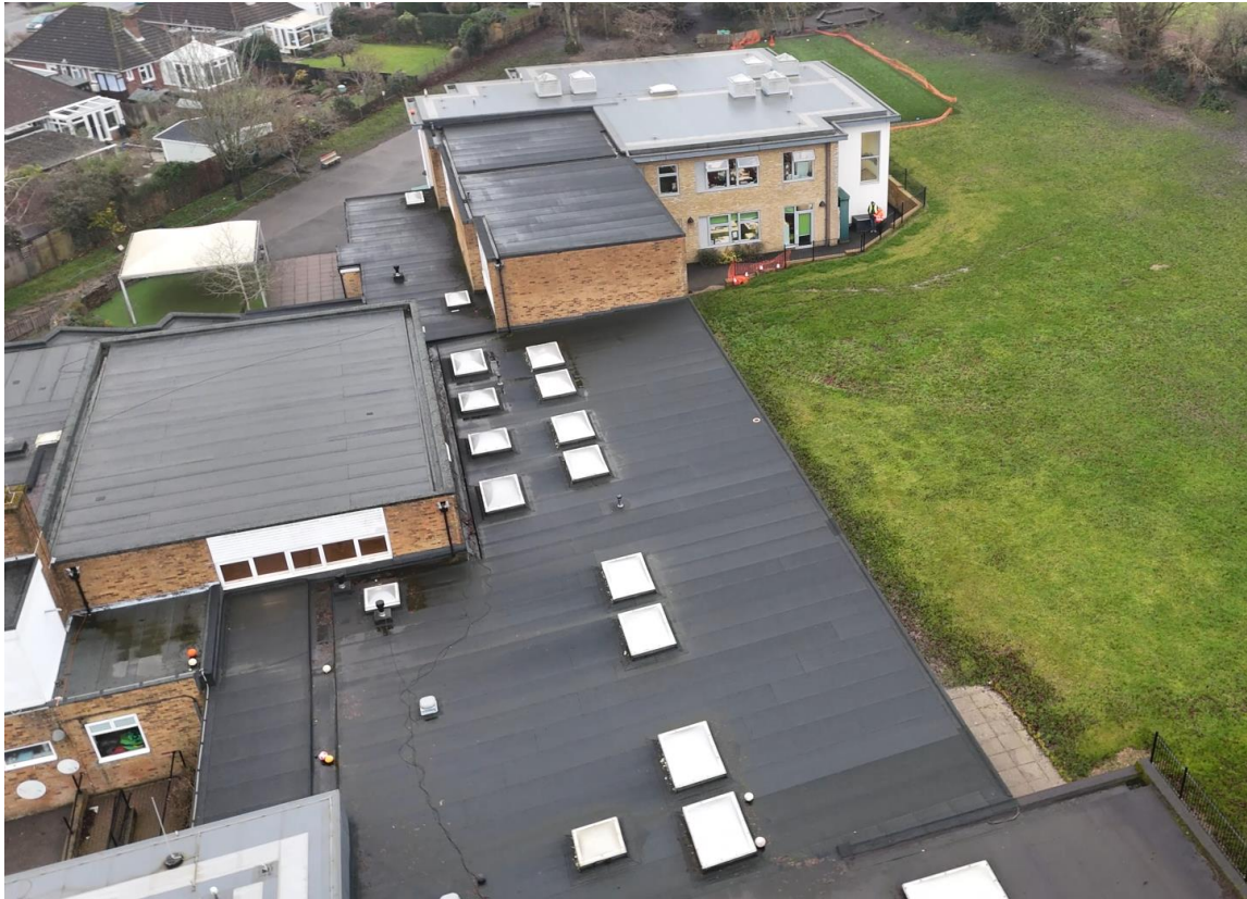
5.6: Image 5: Aerial view to centre of site
