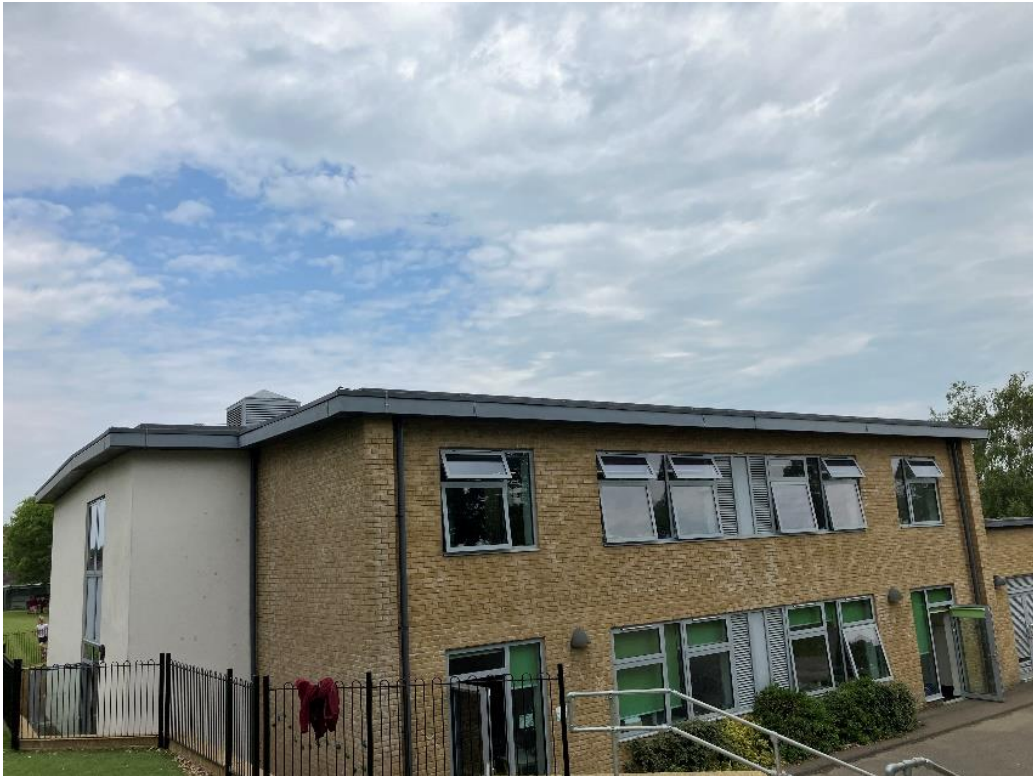
4.5: Image 3 – Ground view from South East of building
