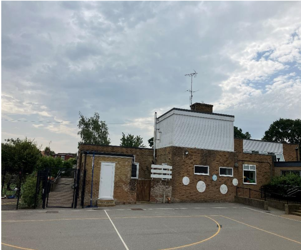
4.9: Image 7 - Ground view from North West of Building
