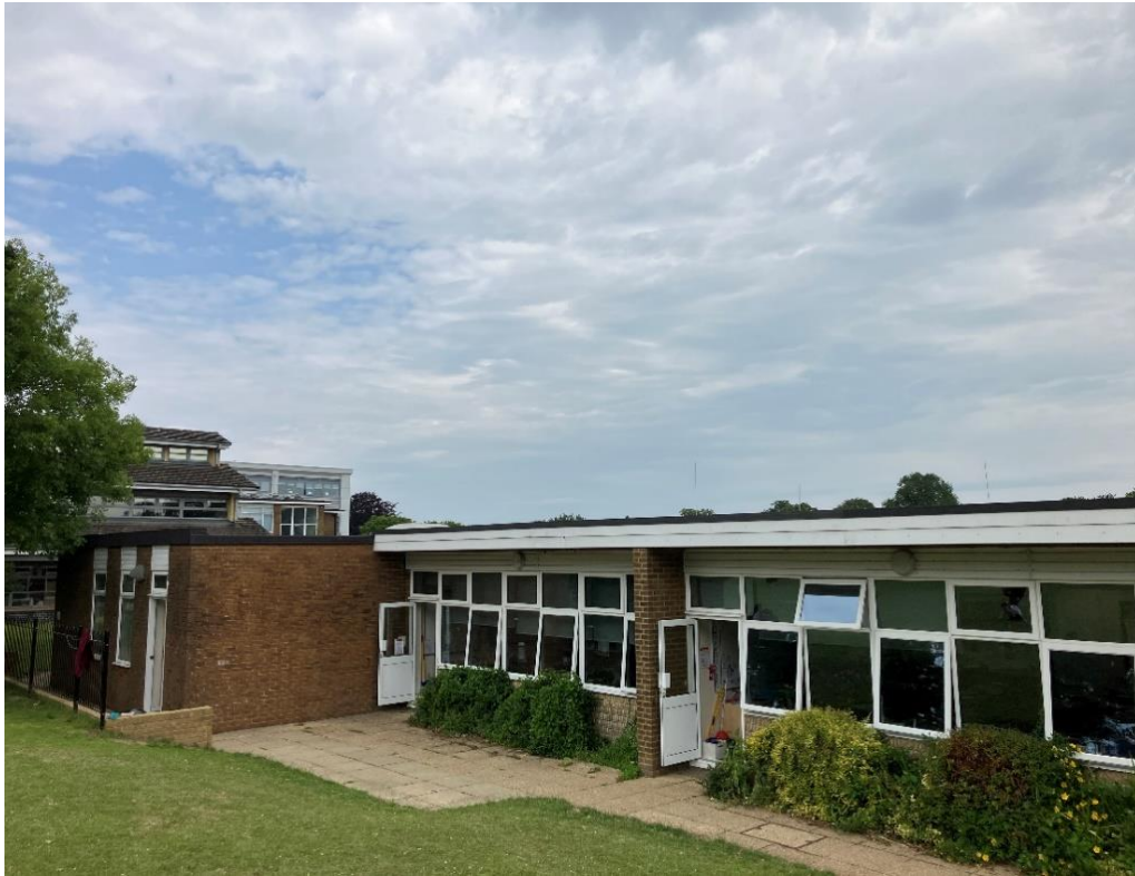
4.7: Image 5 - Ground view from South of building
