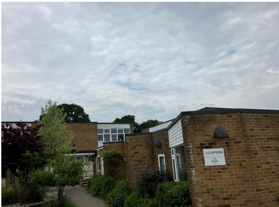
4.4: Image 2 – Ground view from North East of building
