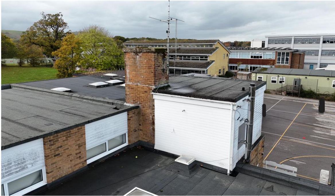
5.2: Image 1 – Arial view of front elevation
