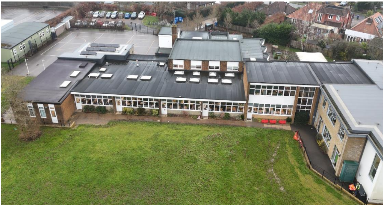
5.5: Image 4 - Arial view to south of site
