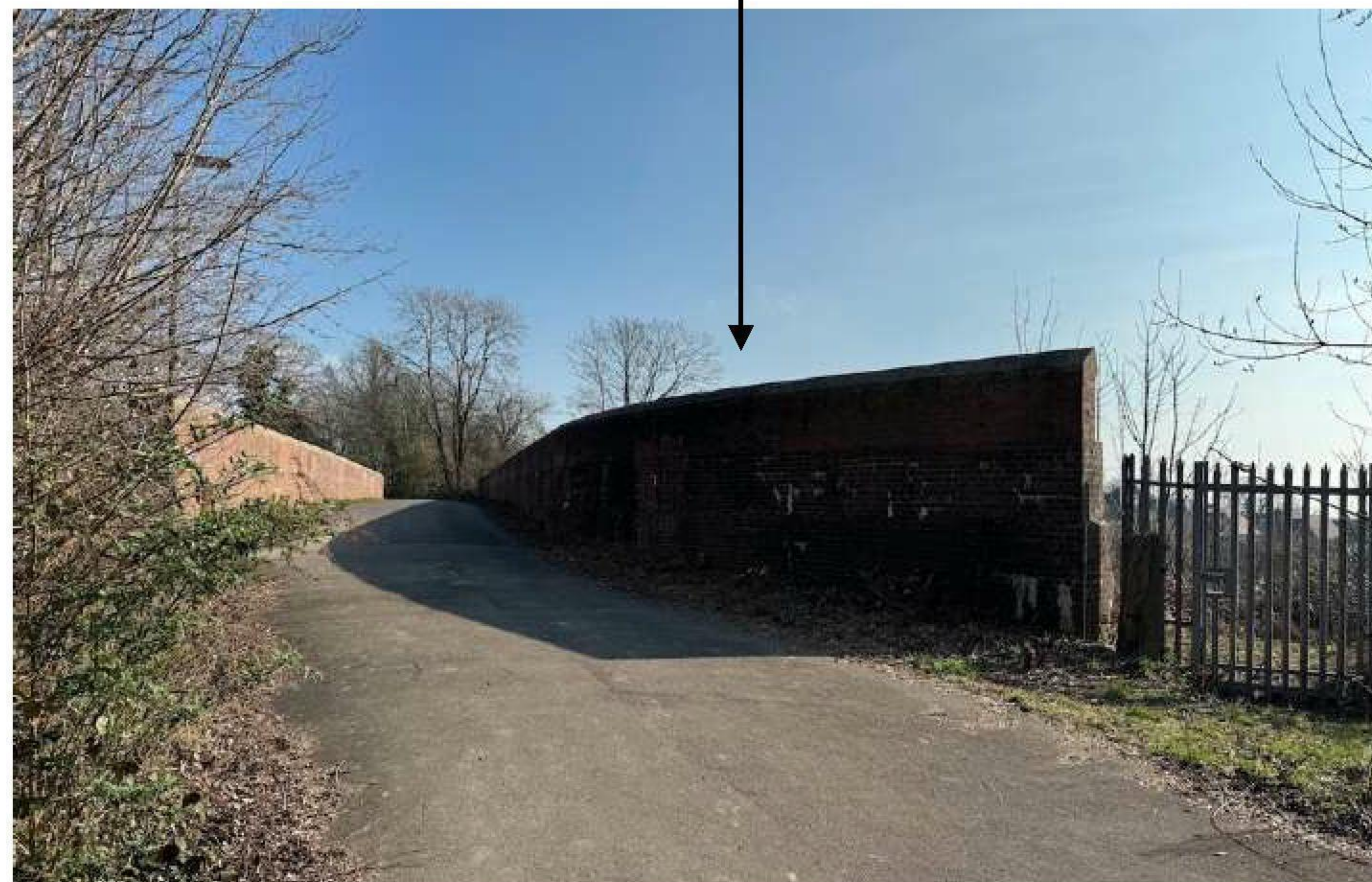
VIEW F - VIEW FROM OLD ROCKY LANE BRIDGE
