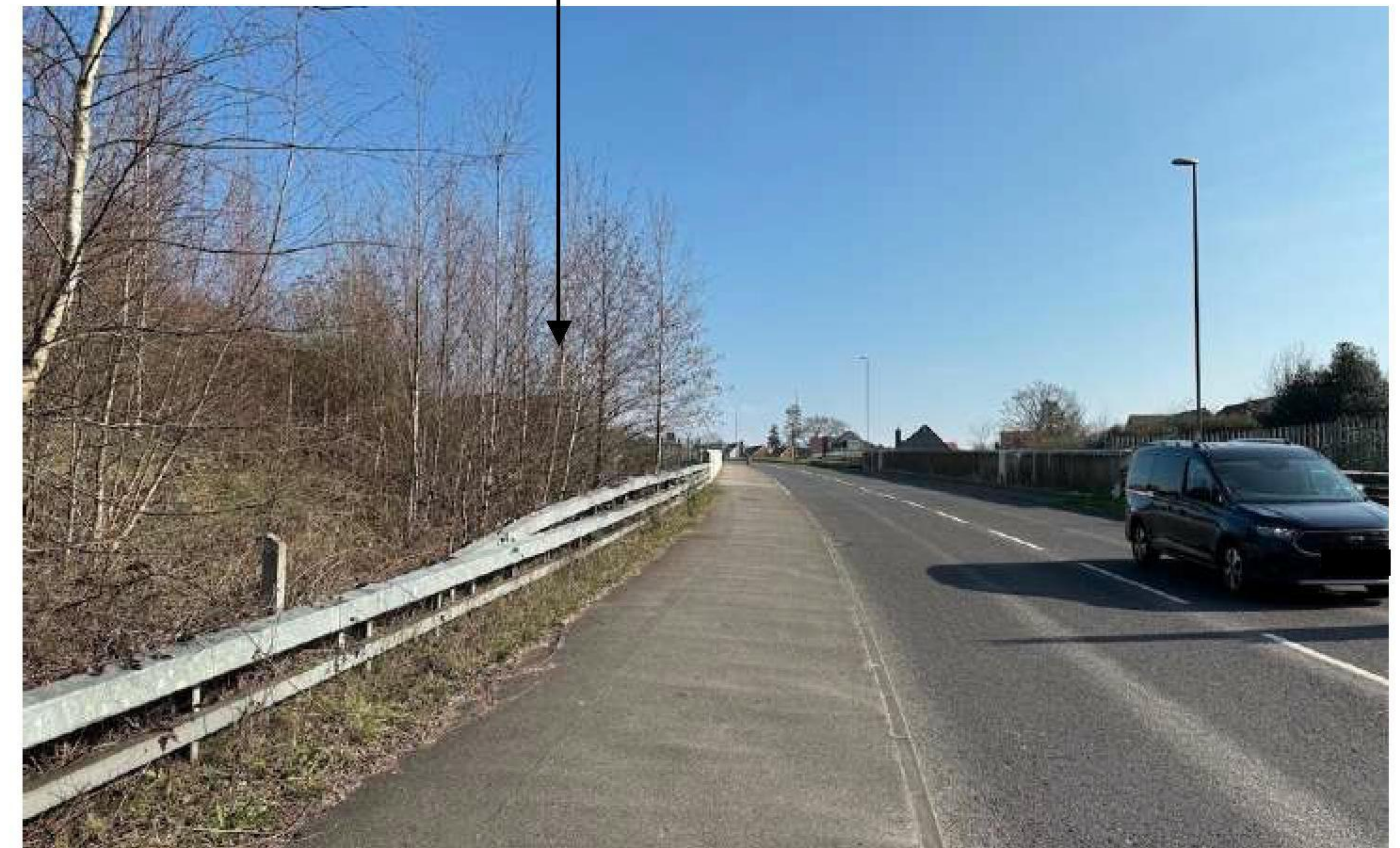
VIEW C - EXISTING VIEW FROM SOUTH-WEST ALONG ROCKY LANE
