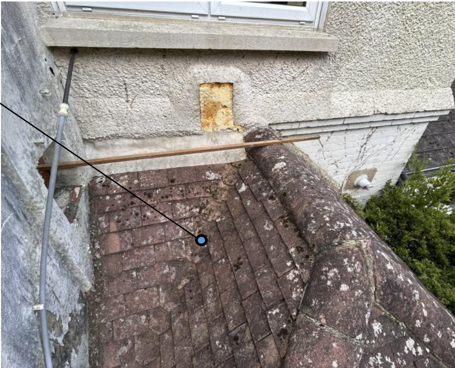
View of hipped extension roof adjacent to stairs, from above. The hip valley is visible in the image where the roof returns against the side of the staircase; this is to be removed and the roof straightened back to the rear elevation
