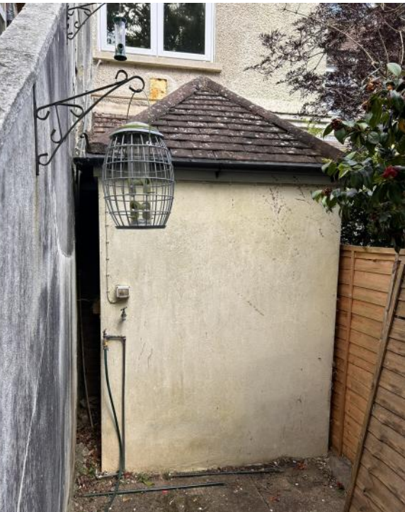
Rear view of hipped extension from ground level.
