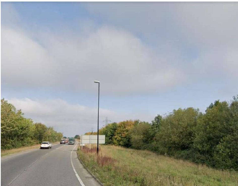
Photograph 5: View looking northwest along the A2300.
