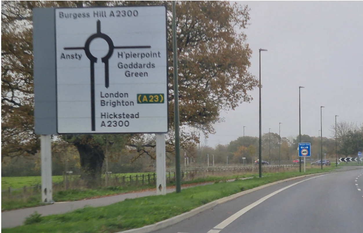
Figure 16: Example of shared use footway passing beneath large sign.
