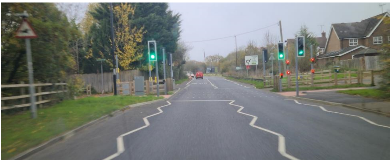
Figure 11: Existing A273 Carriageway, looking north at Gatehouse Lane Pegasus crossing
