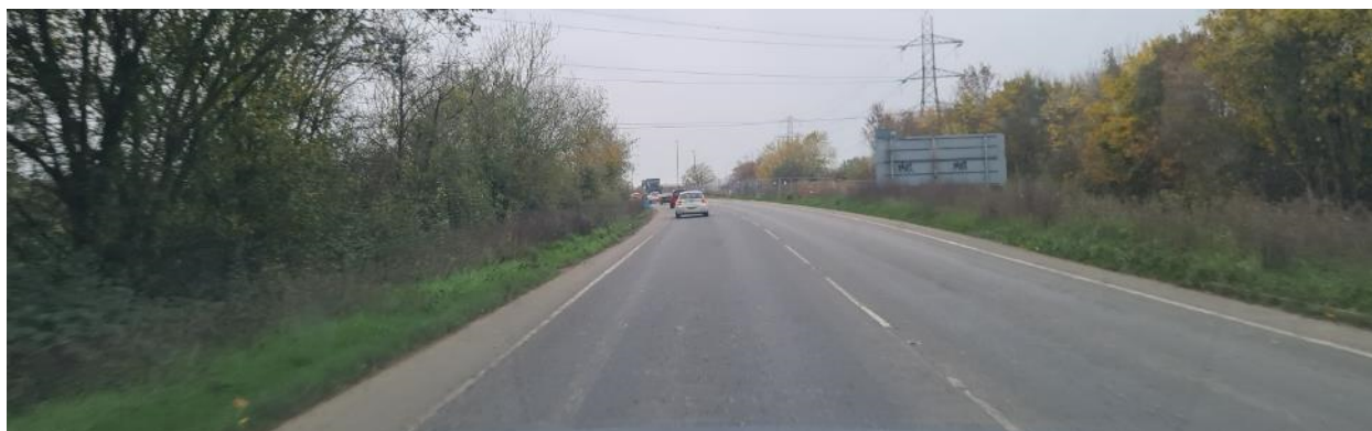
Figure 4: Existing A2300 Carriageway, looking west near the Triangle Roundabout
