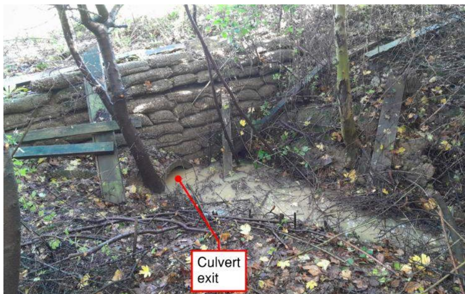
Figure 14: Photo showing the downstream end (exit) of the A2300 culvert
