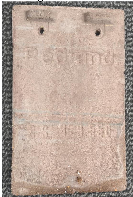
Existing Roof tile rear face
