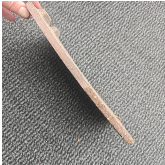
Existing Roof tile profile
