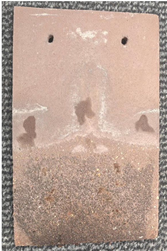
Existing Roof tile front face
