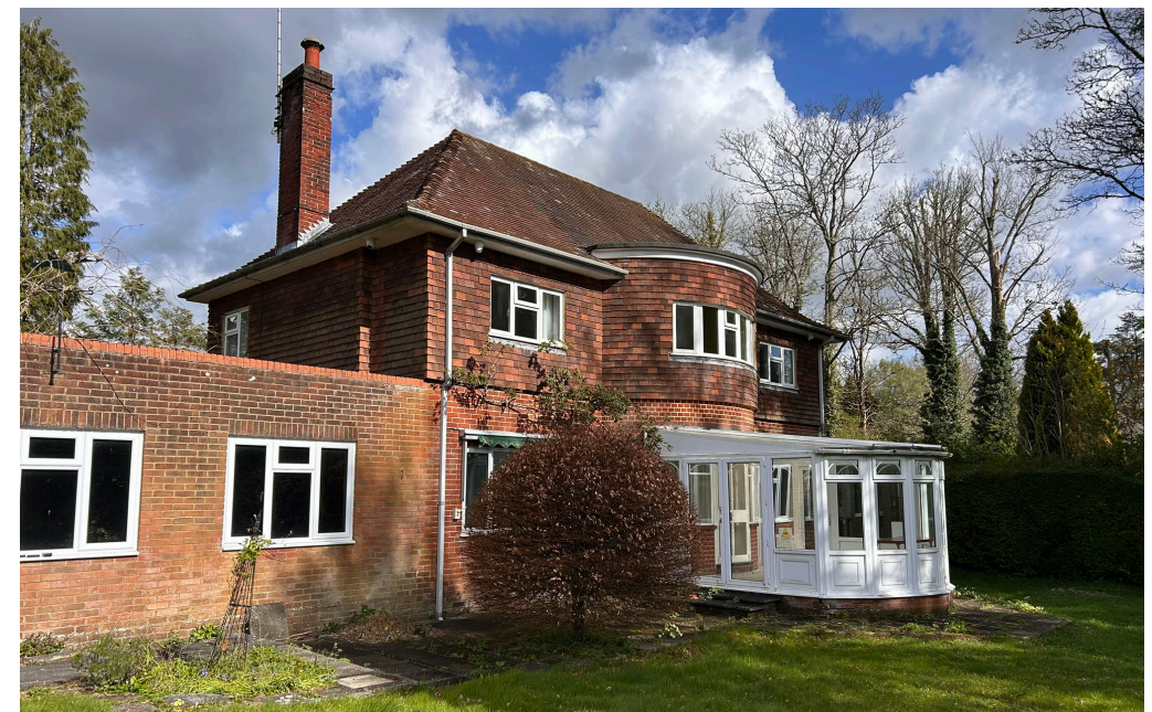
View of rear of Ty Gwilym with the flat roofed garage in the foreground.
