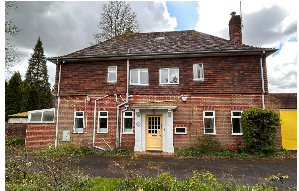
View of front of Ty Gwilym, with Utility on the left and double garage just visible on the right
