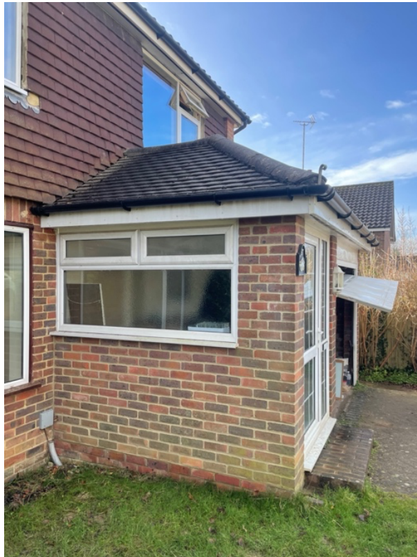
View looking south showing porch & garage
