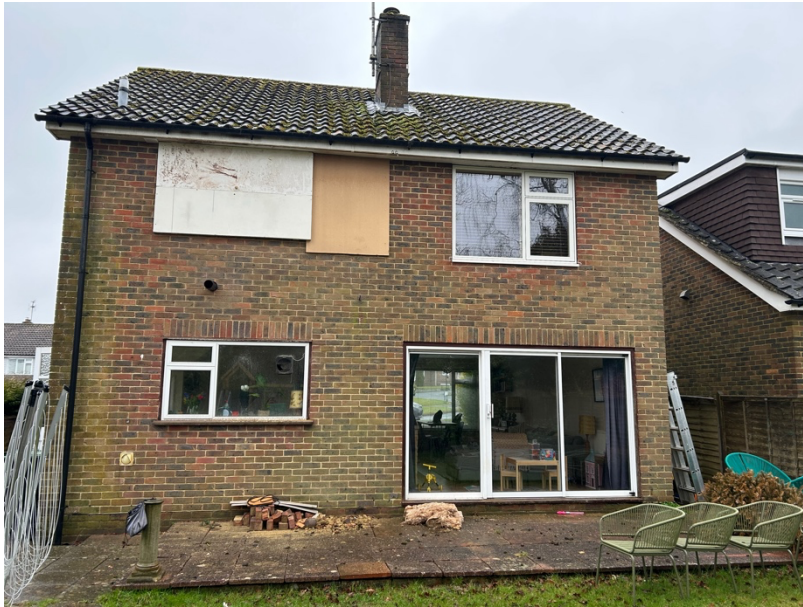
View looking north east showing rear elevation
