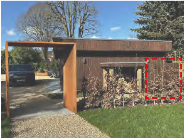
Recent photographs of the irrigation tank enclosure
