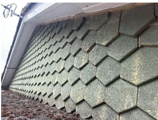
Photograph 3. Hanging tiles on southern elevation and southern gable end.
