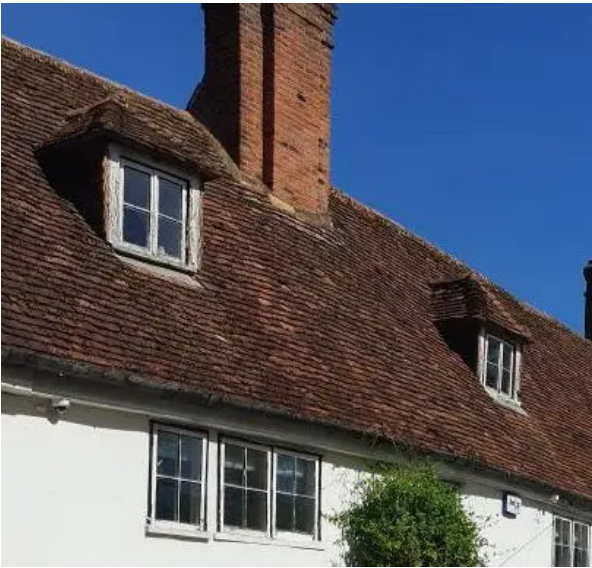
Traditional hipped dormer with flush timber casement windows and tile hanging to dormer cheeks
