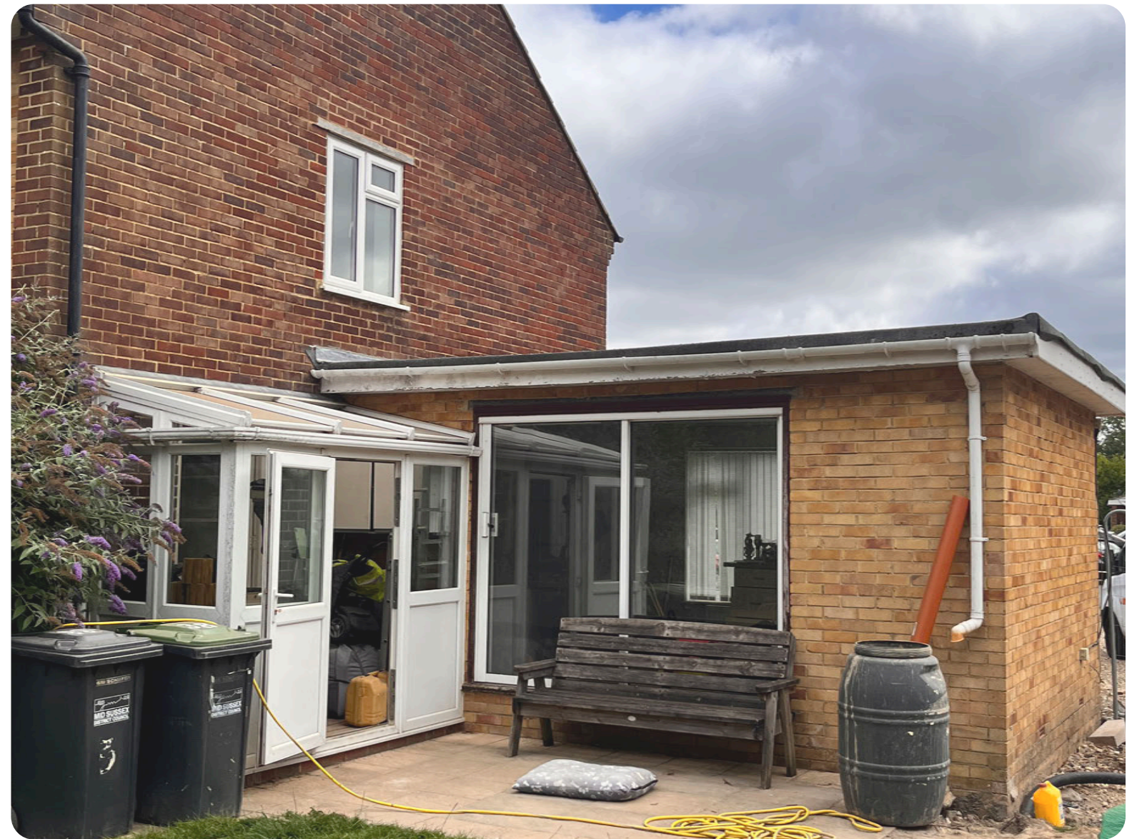
Existing single storey side extension and conservatory to be demolished
