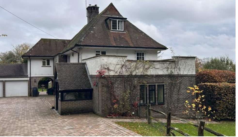
Side West entrance view of existing house with balcony in the foreground. The existing Master Bedroom is to be extended by building over the balcony.
