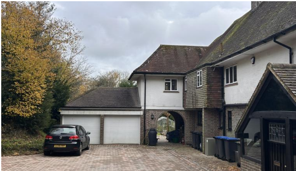
Side West entrance view of existing attached double garage.
