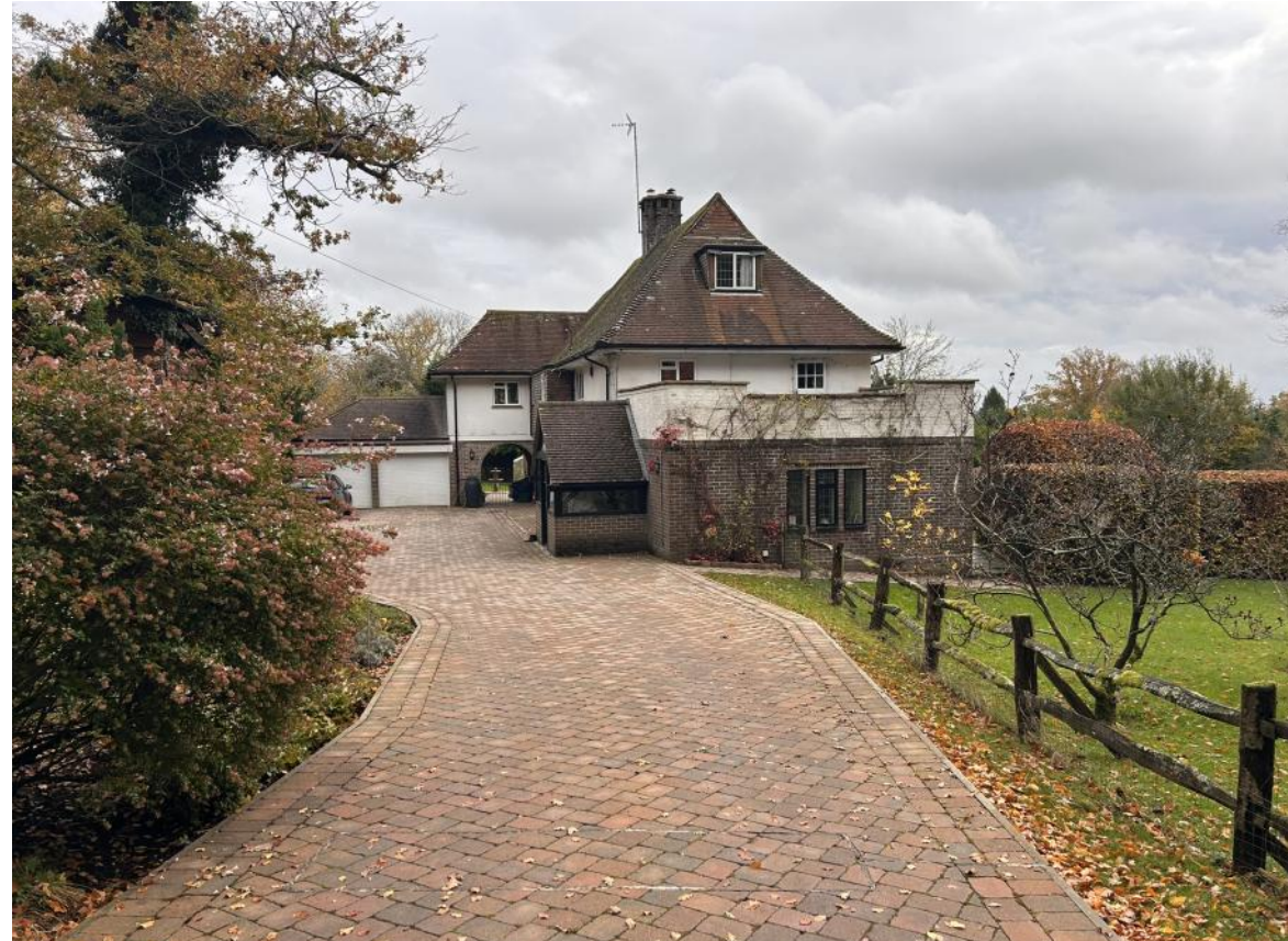
LANDFALL HOUSE, SANDHILL LANE, CRAWLEY DOWN
