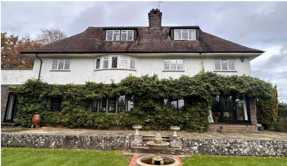
Front South view of house from garden. Master bedroom is at first floor on the left side with balcony just visible.
