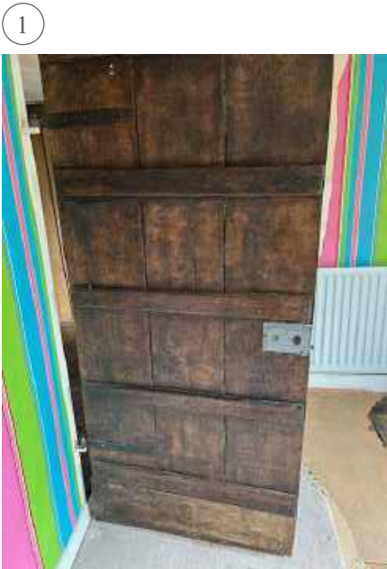
Existing timber door (to be reinstated and fixed shut)
