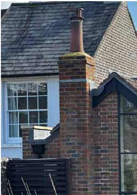
Recent photograph of parapet wall detail
