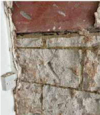
Blockwork construction underlying the exposed timber stud wall with stonework nogging
