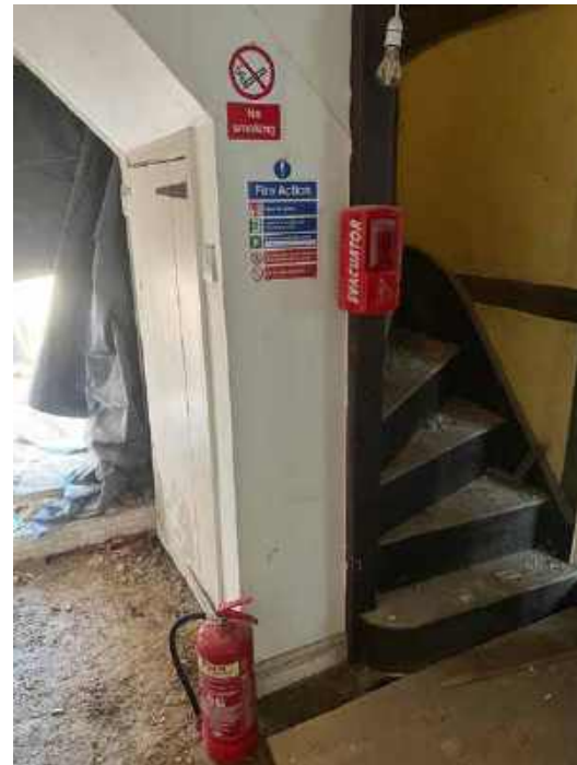
Staircase during demolition works
