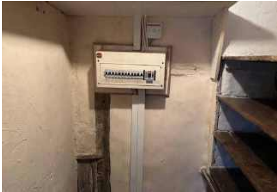
Pre-construction photograph of original wardrobe
