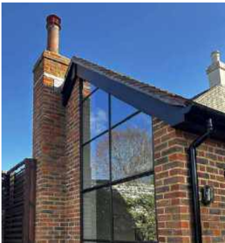
‘As-built’ bake house chimney with lead waterproofing dressing
