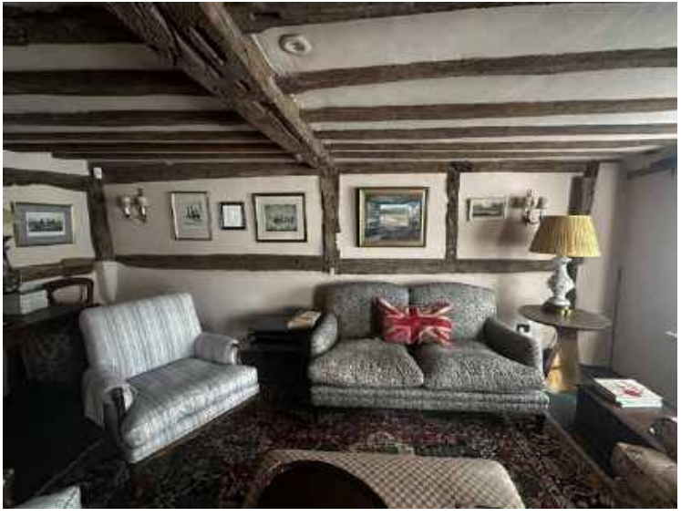
Ground floor living room - removed chimney breast and wall and ceiling made good
