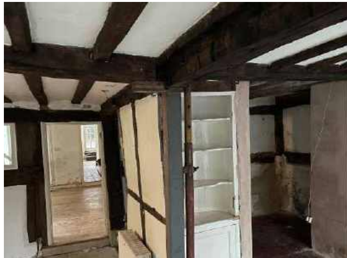
Internal wall and steel beam before removal
