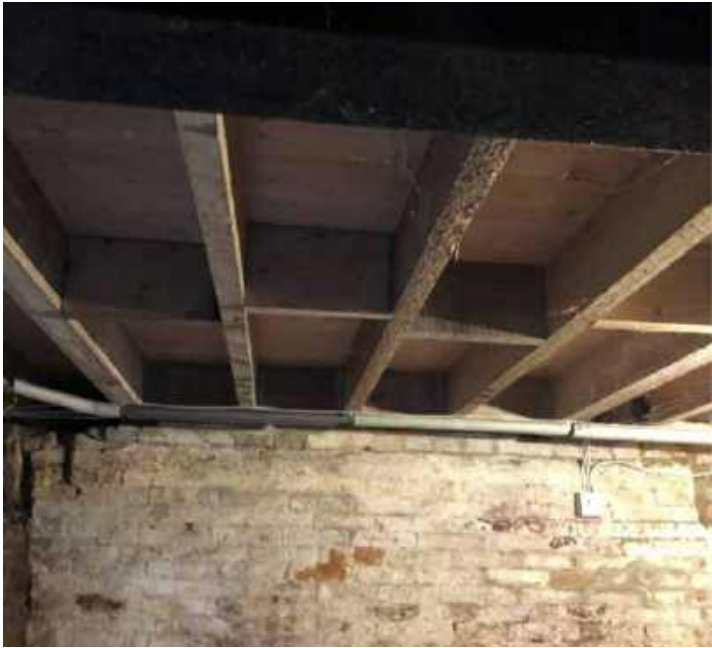
New softwood joists, basement
