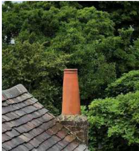
Original bake house chimney
