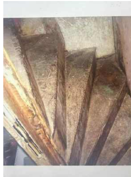
Staircase during demolition works
