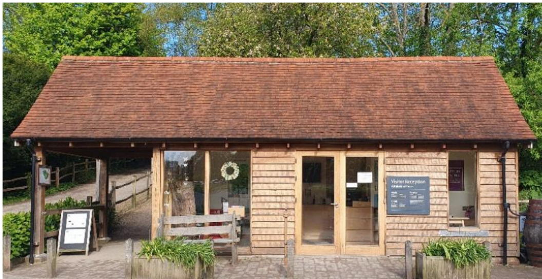
Photo 1: External finish and materials of existing VR building, Standen car park. Source: Baird Design.
