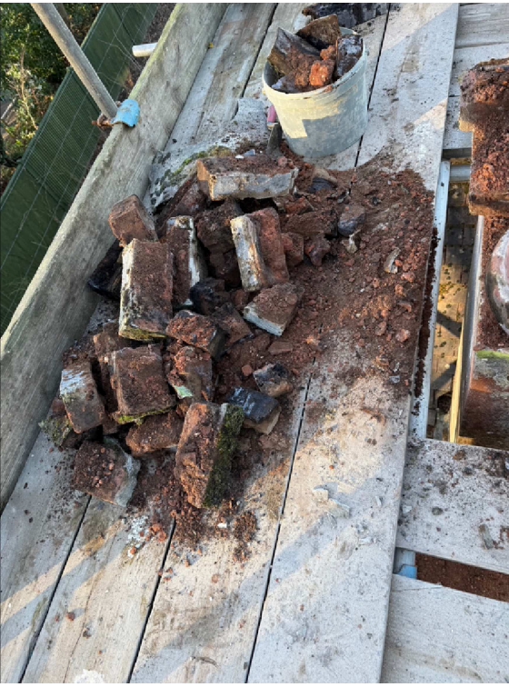
Poor quality of the masonry as removed.
