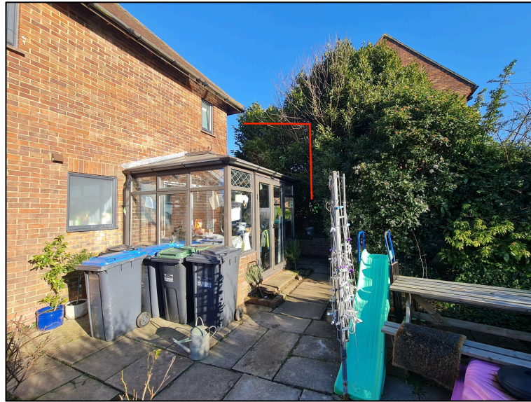
Figure 1: Red line indicating small section of T2 to be removed.
