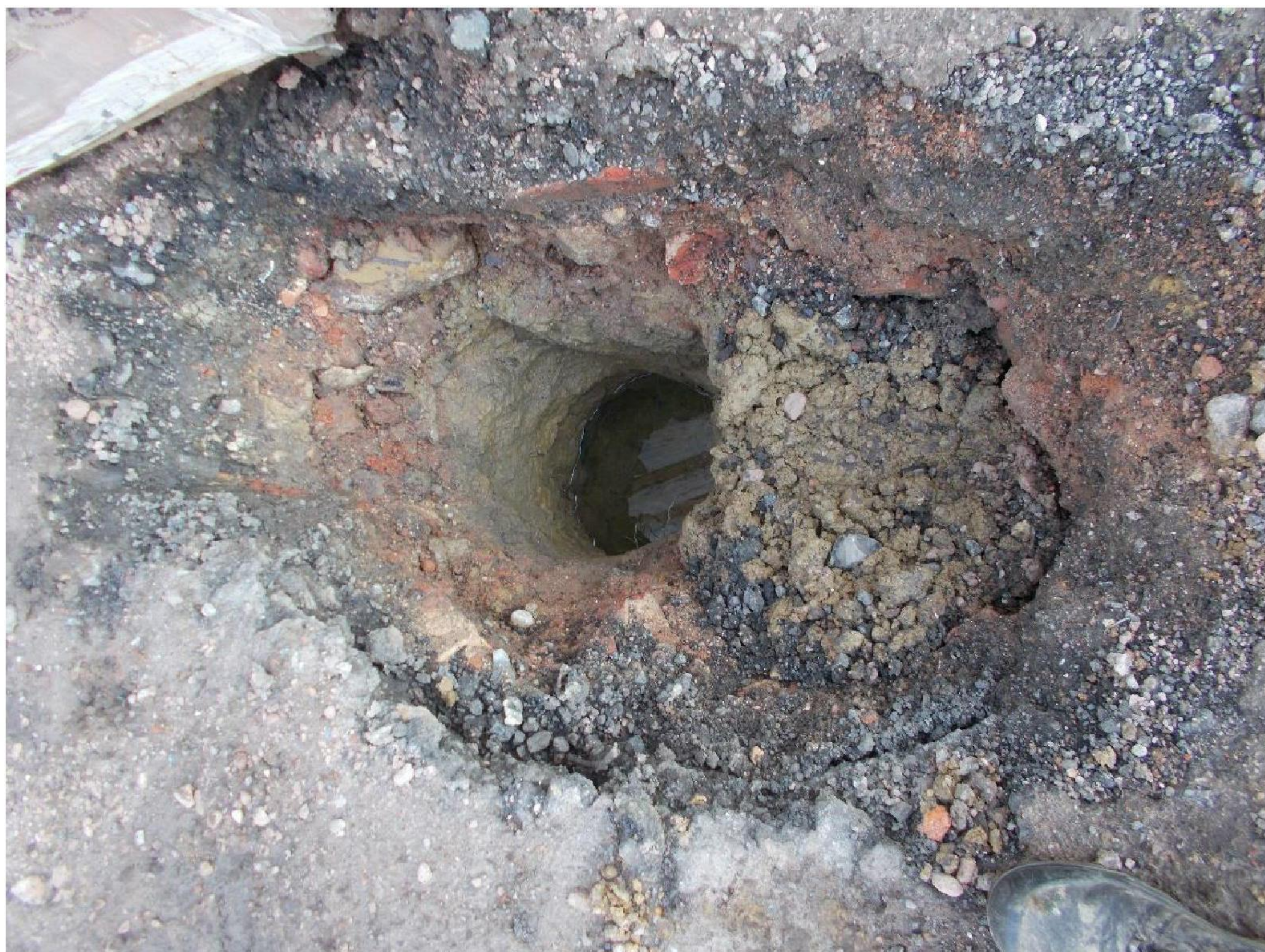
Photo 2: Trial hole excavation. Note clay close to the surface.
