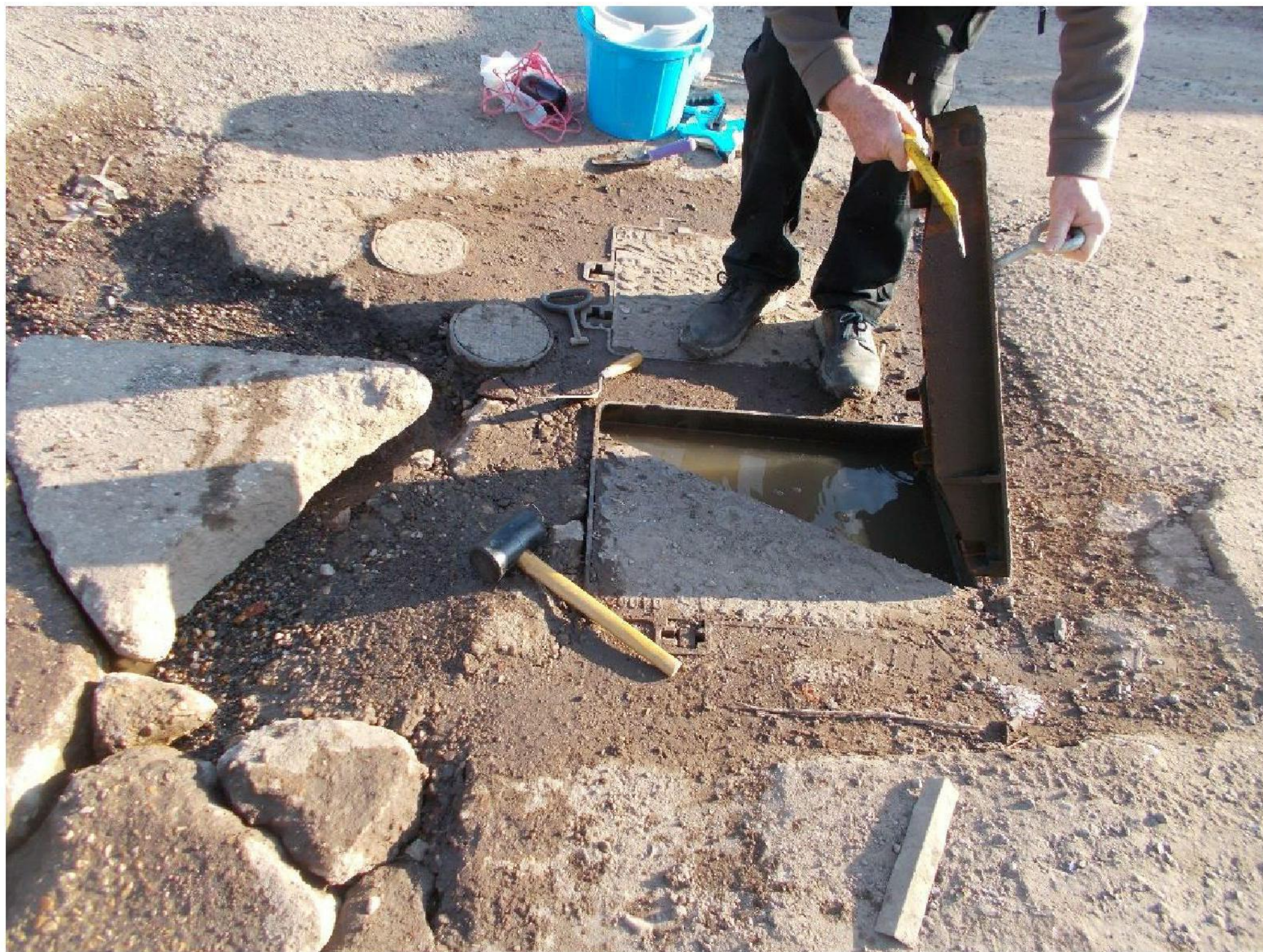
Photo 1: Chambers in the site entrance
