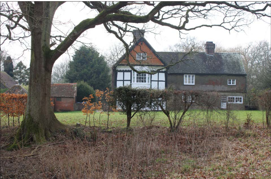
PHOTOGRAPH – VIEWPOINT S6 VIEW OF THE NORTHERN ELEVATION OF THE GRADE II LISTED THE PLACE.
