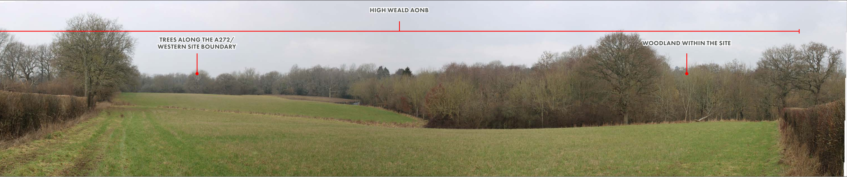
PHOTOGRAPH – VIEWPOINT S10 VIEW FROM THE CENTRAL PART OF THE SITE, LOOKING WEST TOWARDS THE HIGH WEALD AONB. THE WOODLAND WITHIN THE SITE AND THE TREES ALONG THE A272 SCREEN VIEWS OF THE GROUNDPLANE OF THE AONB.
