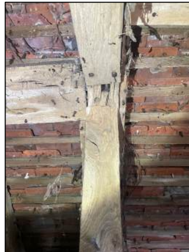
Photograph 4: A mortise and tenon joint within building B1.
