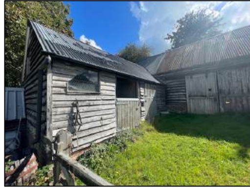
Photograph 12: Buildings B3 and B4 from left to right.
