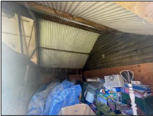
Photograph 13: The internal of the western extent of building B4.
