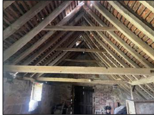
Photograph 6: The upper level of building B1.
