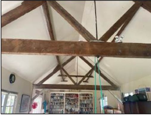
Photograph 11: The internals of building B2.
