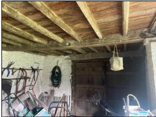
Photograph 7: The lower level of building B1.
