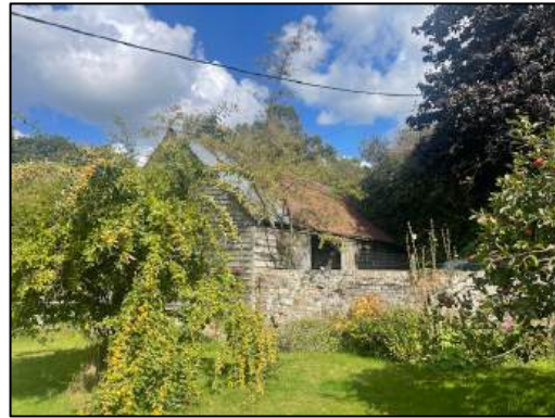
Photograph 14: The south-eastern elevation of building B4.
