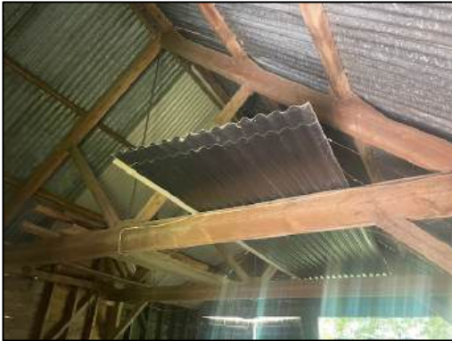
Photograph 15: The internal of the eastern extent of building B4.
