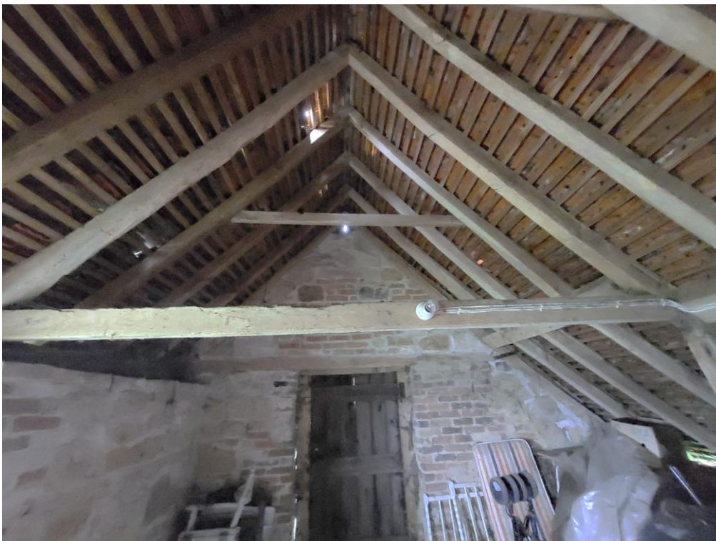
Photograph No. 04 – Internal Inspection of B1, looking north
