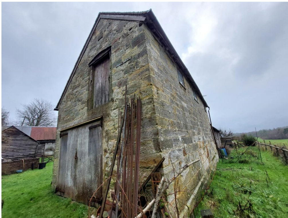
Photograph No. 02 – North and west aspects of Building B1.
