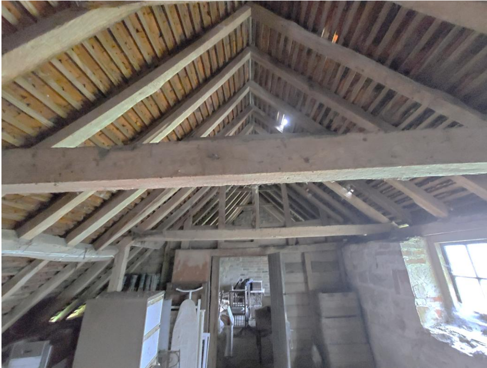
Photograph No. 03 – Internal Inspection of B1, looking south.
