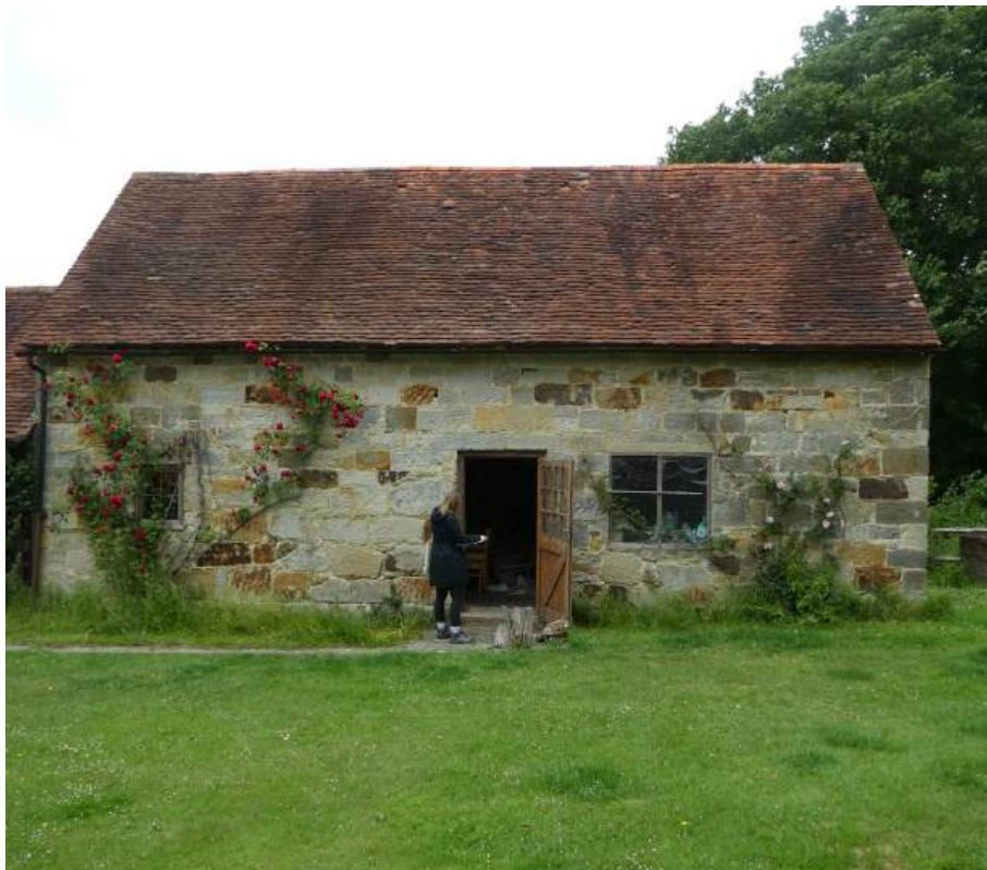
1. View of Stone barn from courtyard
