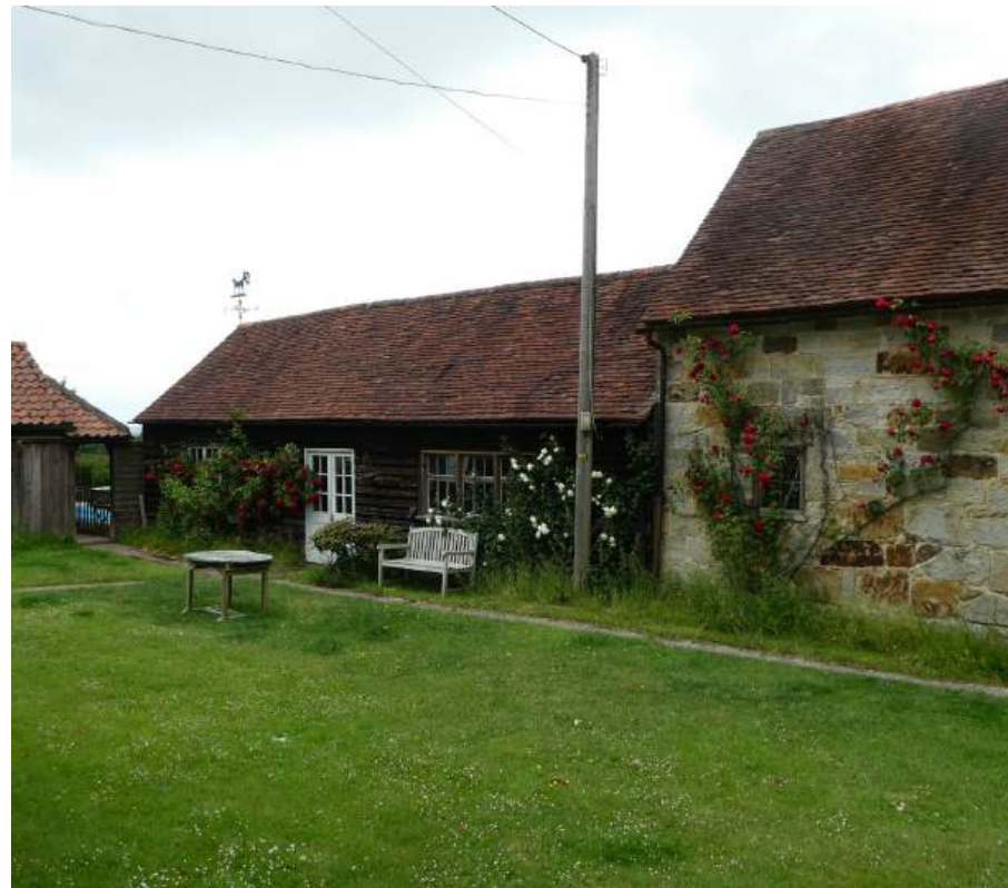
2. View of Timber clad barn from courtyard
