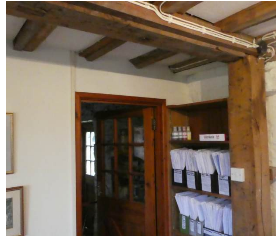
3. Stone barn structure to ground floor
