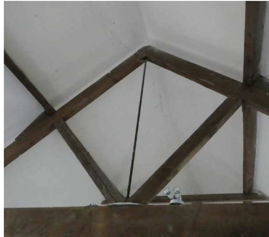
2. Roof structure to timber barn
