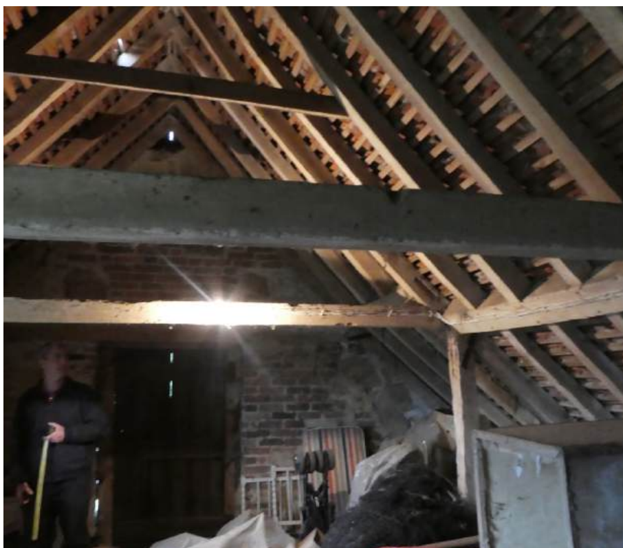
4. Stone barn roof structure
