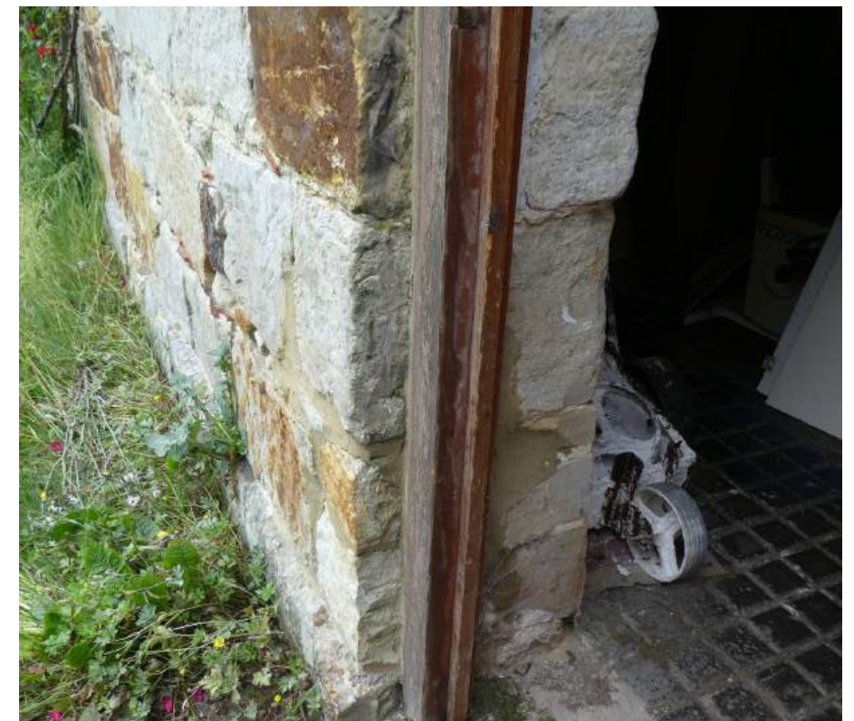
6. Stone barn wall build-up
