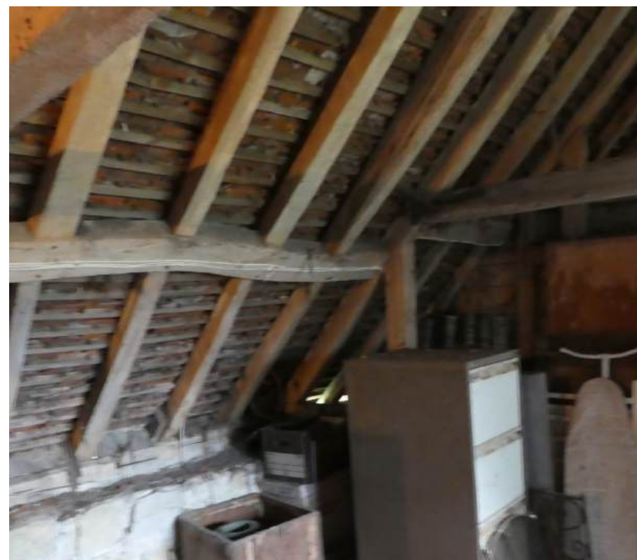
5. Stone barn roof structure
